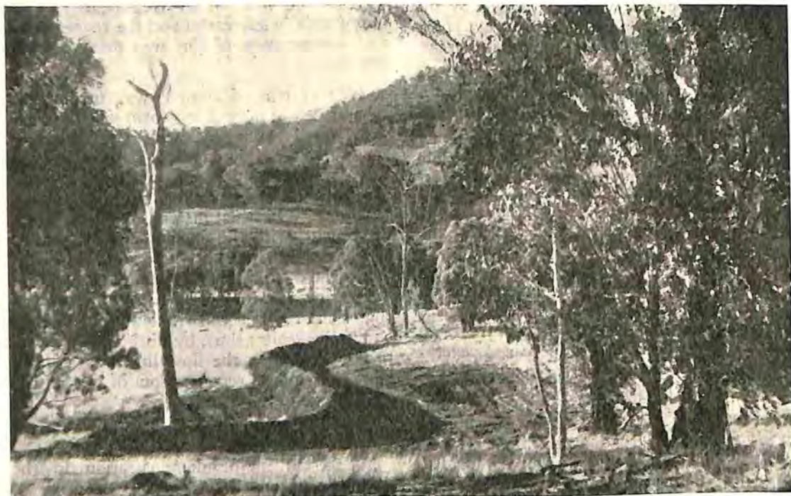
Fig. 4.—A diversion bank takes surplus water to dams.
