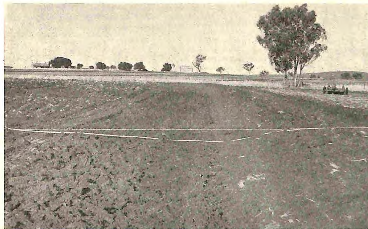
Fig. 3.—A graded bank on a 6 per cent. slope with gentle batter into the channel.
