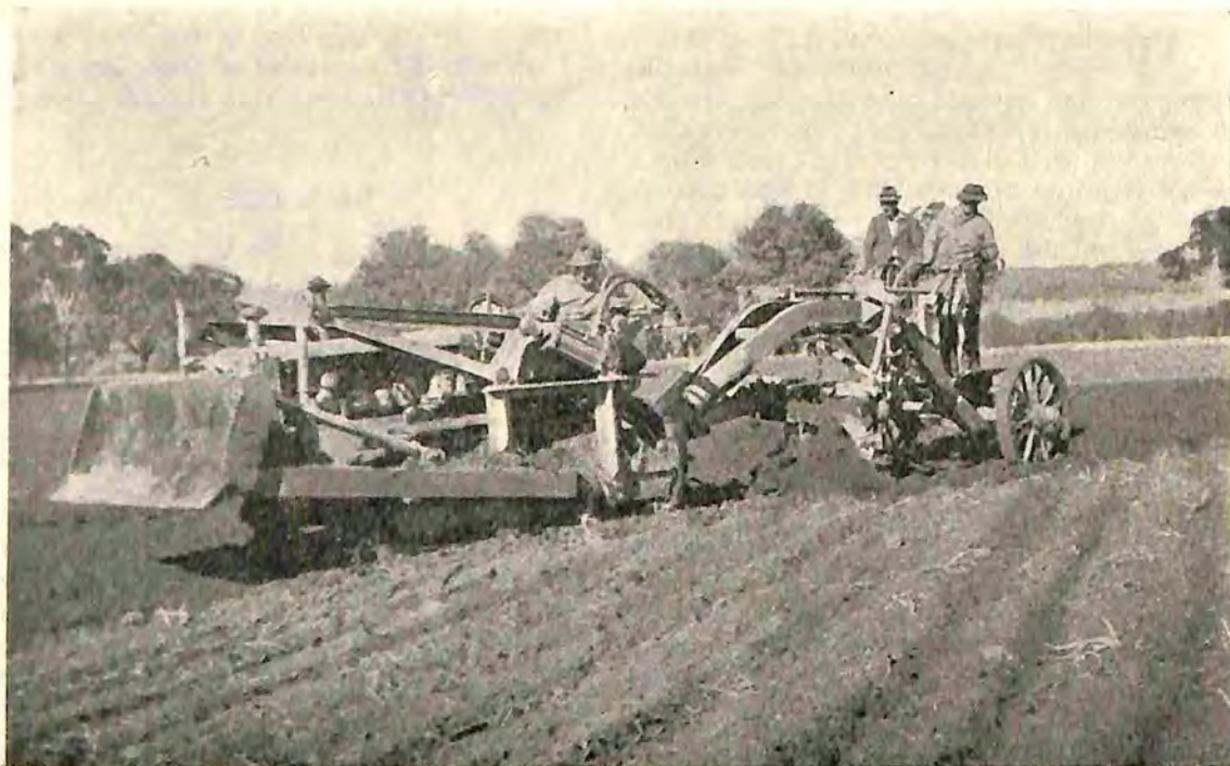
Fig. 3.—Soil Conservation Service plant at work on Roseneath, Inverell.
