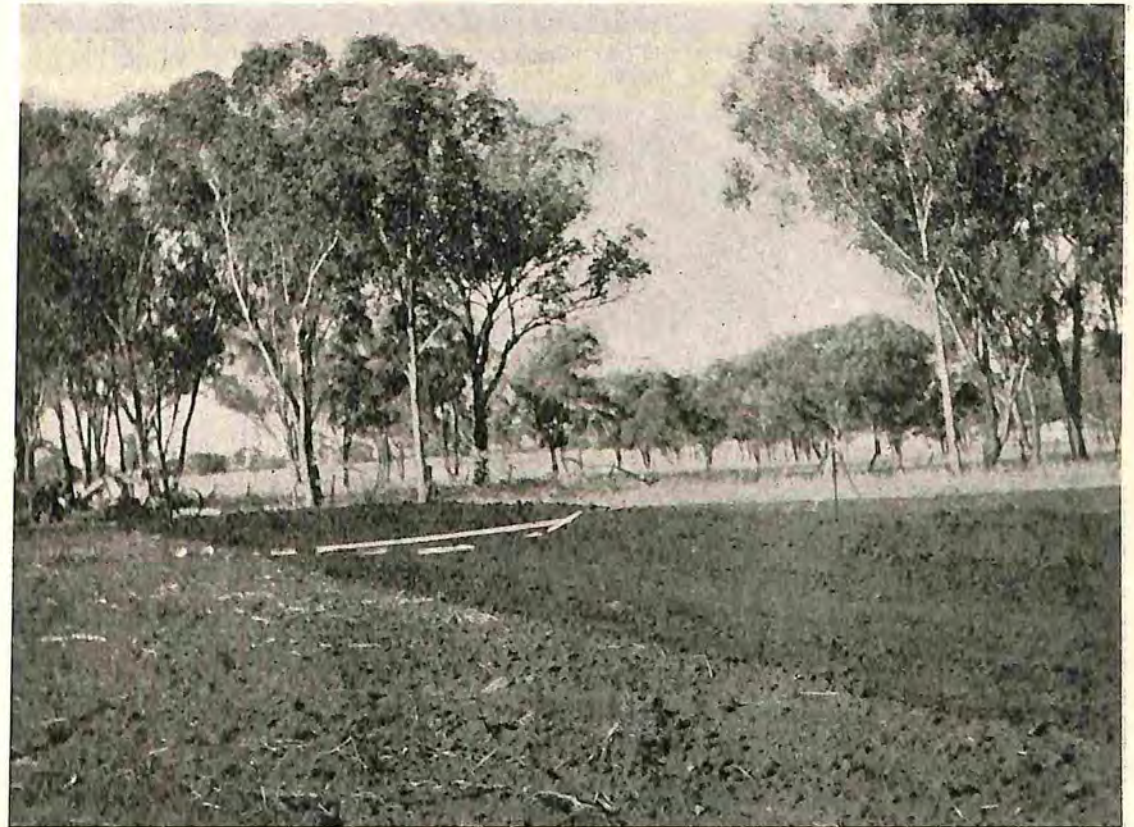
Fig. 4.—Broad-based banks discharge into safe timbered areas.
