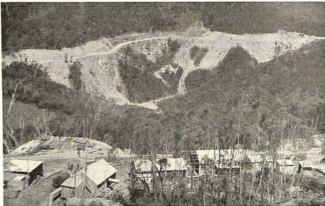
Fig. 8.—Serious erosion hazard created during construction of the Snowy Valley road near Munyang. (Photo S.M.H.E.A.)
