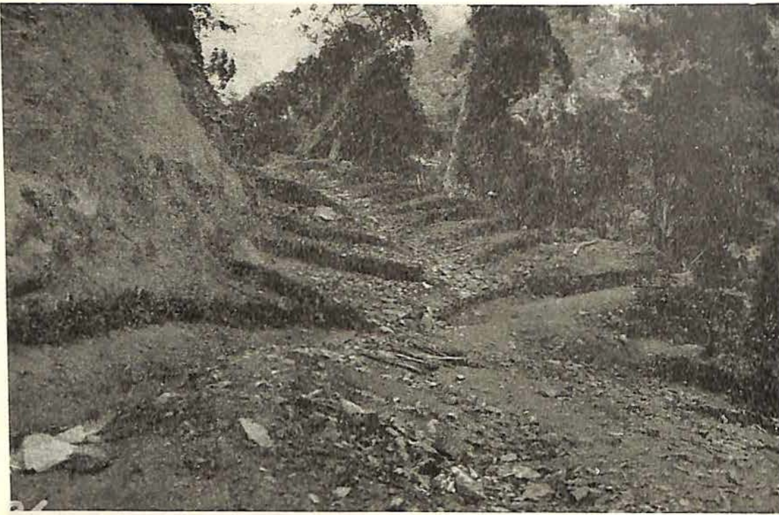
Fig. 14.—Wattled fences and a stone-pitched waterway in the early stage of revegetating a disused track. (Photo. S.M.H.E. A.)
