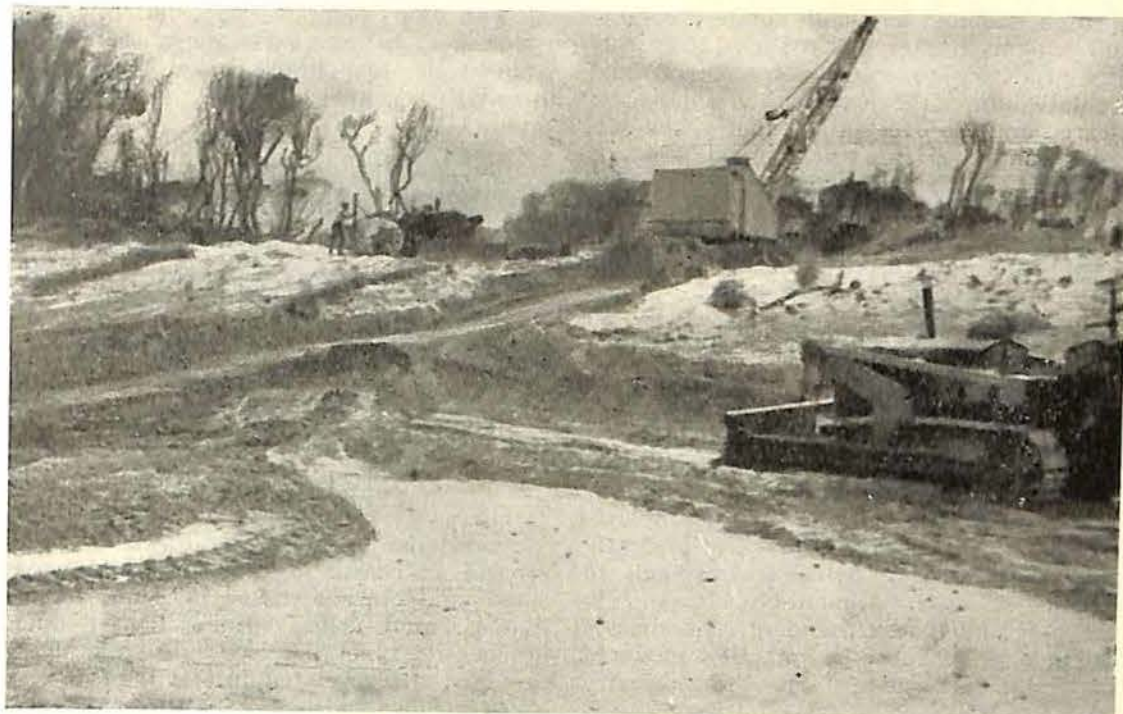
Fig. 1.—CUDGEN. Open cut mining of frontal dune.
