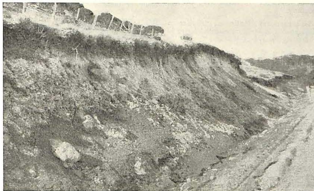
Fig. 2.—Needle ice on a road batter near Kiandra showing typical recession of the slope face.
