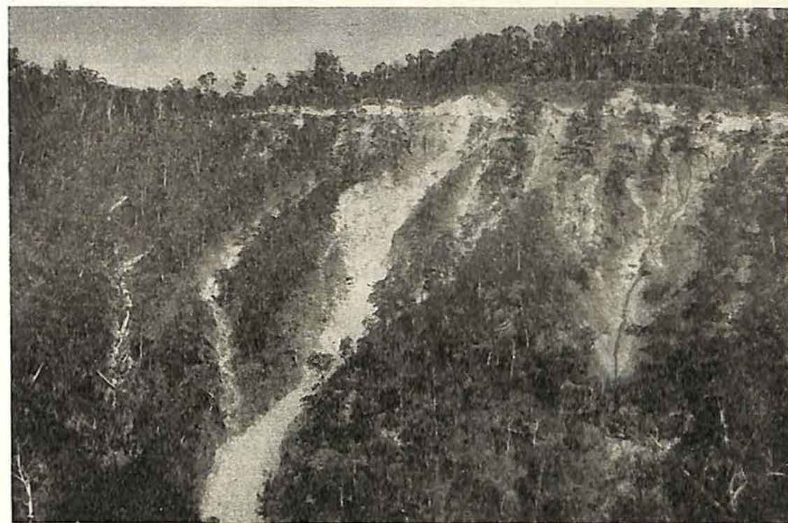
Fig. 7.—Dumping spoil followed by debris slides has destroyed the stability of this slope below Happy Valley road.
