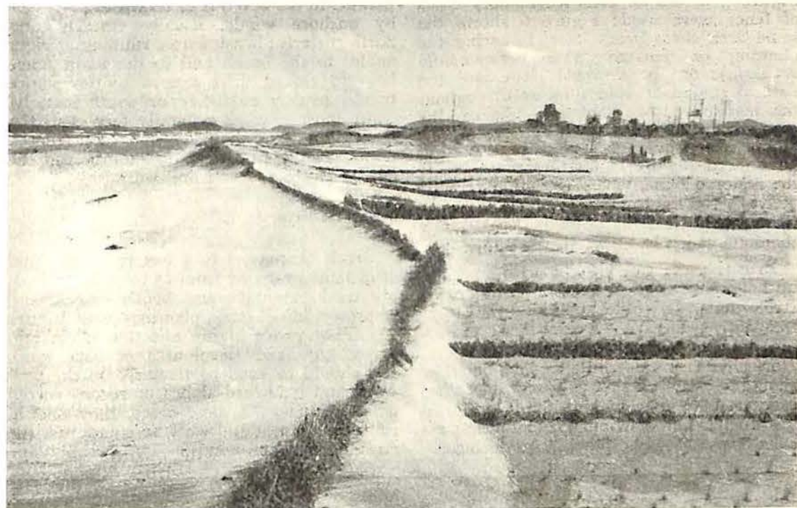
Fig. 7.—CUDGEN. Brush fence and barriers protecting young marram grass plantation; seaward slope not yet treated.
