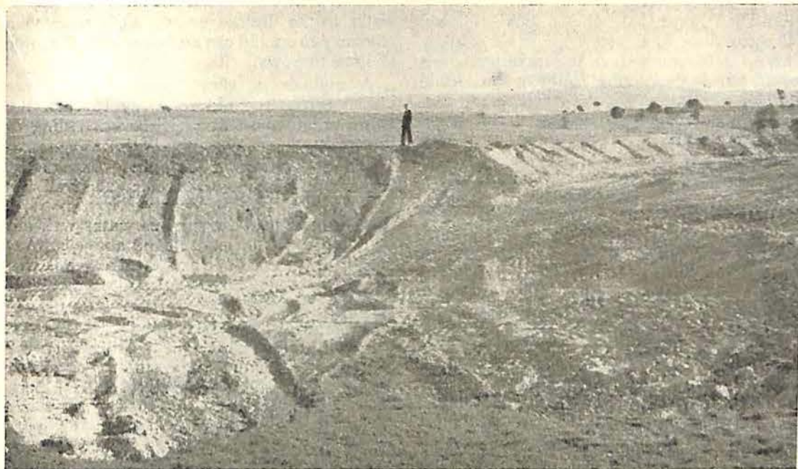
Fig. 3.—The gully check dam at A in Fig. 1, showing massive bank and overflow bank at right.
