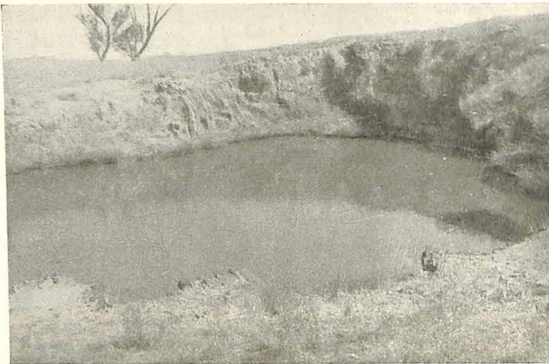
Fig. 5.—This quarry in the Canowindra District, with an estimated capacity of 15,000 cubic yards, has been used as an outlet for graded banks.
