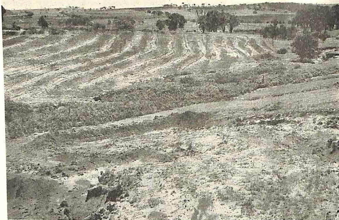
Fig. 1.—Mechanical soil conservation measures must be followed by vegetative cover to achieve complete stabilisation.
