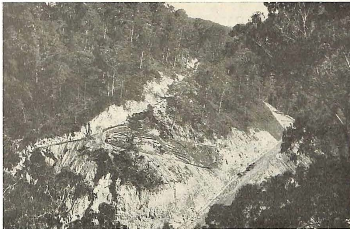
Fig. 9.—The lower leg of Happy Valley Road with the former access track above. The slopes have been seriously damaged by dumping spoil and opening the lower batter face.
