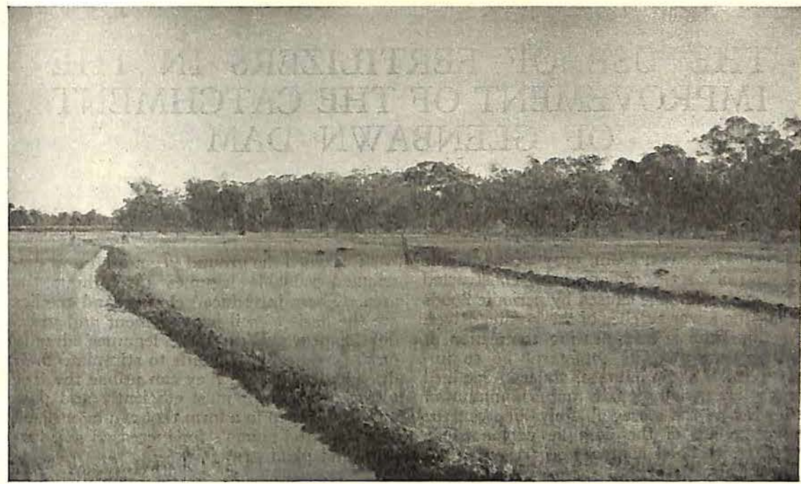
Fig. 6.—Pasture furrows, constructed with farming equipment, retain run-off.
