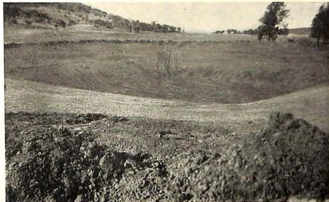
Fig. 2.—Silt dam on the demonstration immediately after completion.
