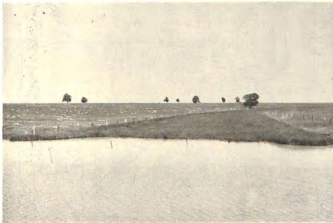
Fig. 2.—A first-class waterway carrying run-off from the south-western part of the demonstration into a dam.
