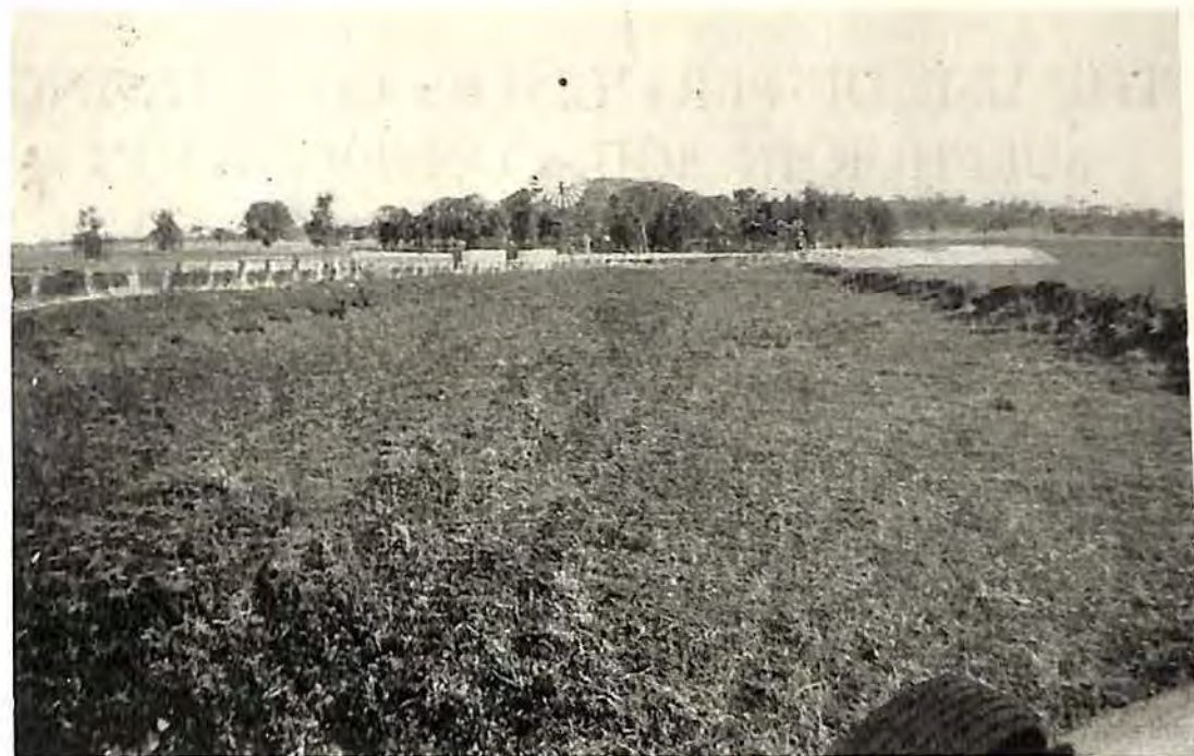
Fig. 5.—Looking up constructed waterway towards silt dam.
