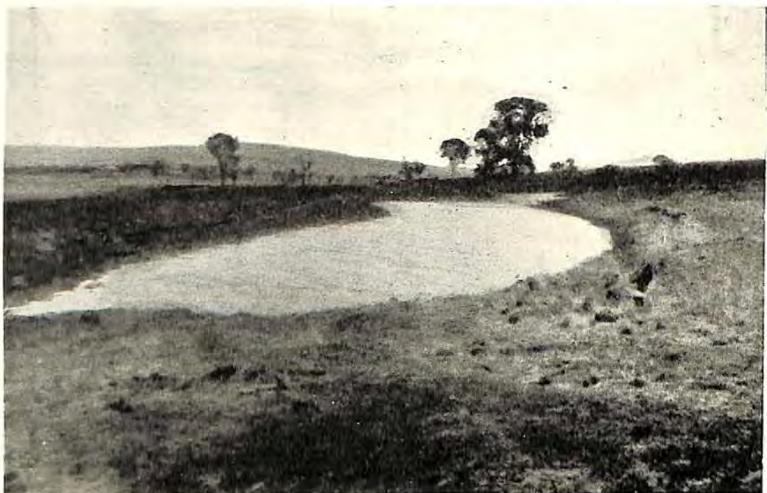
Fig. 4. A park and channel constructed on this principle (see fig. 3.) after heavy rain—outlet in foreground.
