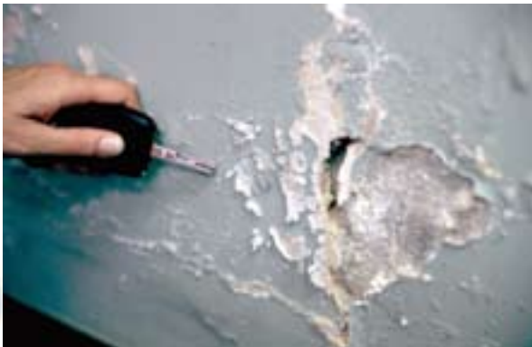
Salt crystals forming under paint on a wall after numerous wetting and drying cycles.
