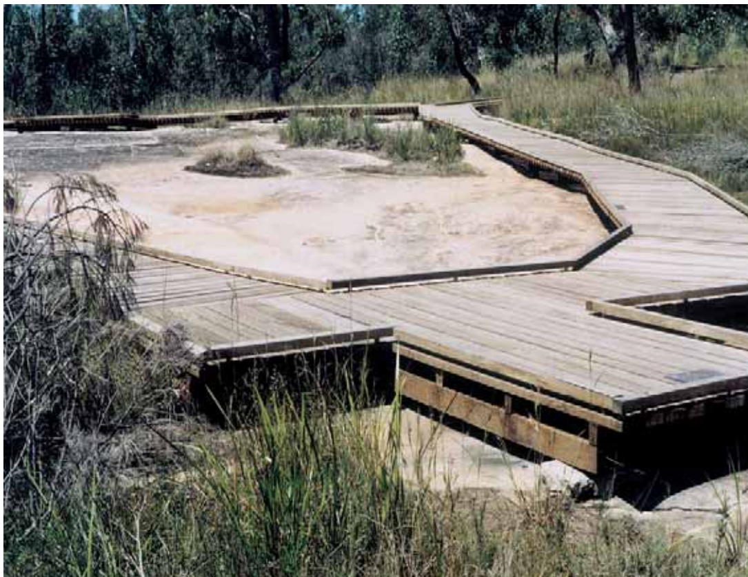
Plate 28. The new boardwalk at Bulgandry. It is designed to sit on the rock rather than being fixed by drilling into the rock.
