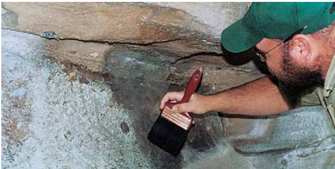
Plate 4: Dry lichen at Gnatalia Creek being removed by dry brushing. This work was carried out in 2002 and followed recent fires.
