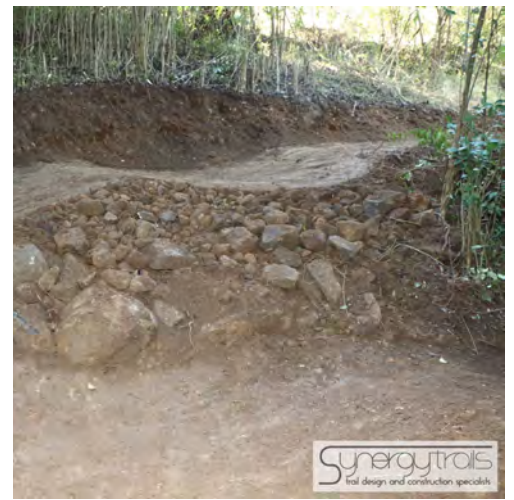
Rolling Dip with Hardened Spill Way
