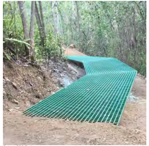
Raised FRP Trail
