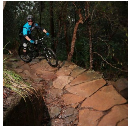
Rock Armoured Berm
