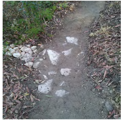
Hardened Spill way with DSR
