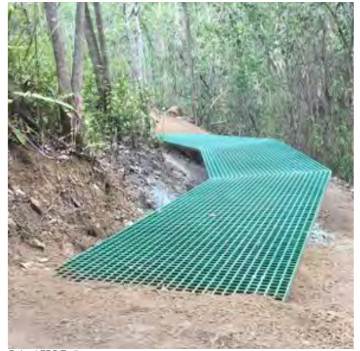
Raised FRP Trail
