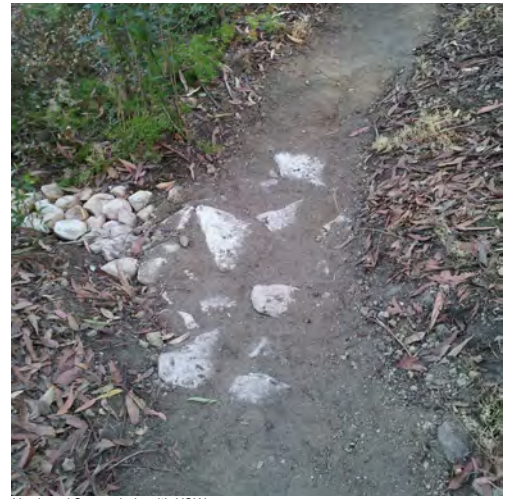
Hardened Spoon drain with HSW
