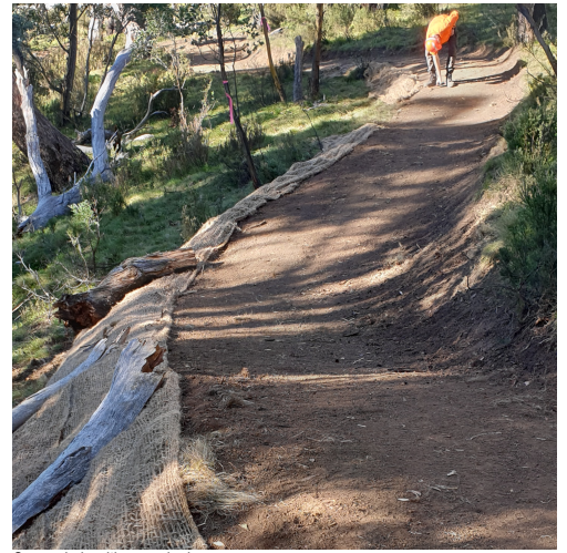
Spoon drain with spreader log
