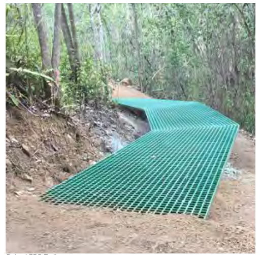
Raised FRP Trail
