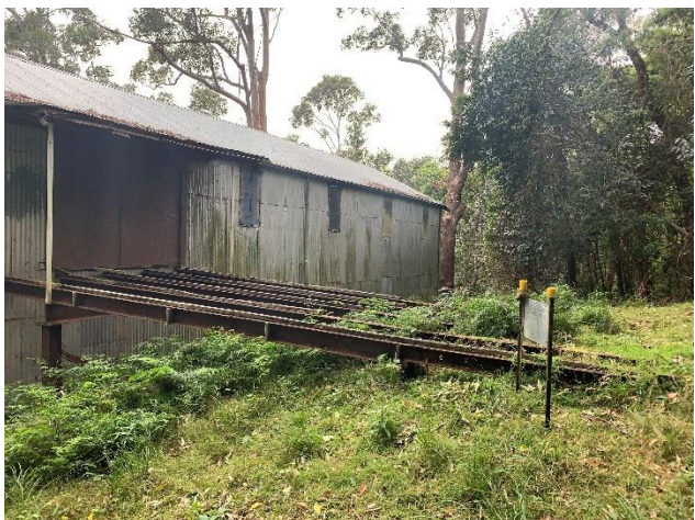
Plate 67: Ramp made of rail girders (Source: Niche)
