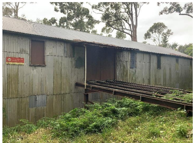
Plate 68: Ramp made of rail girders (Source: Niche)
