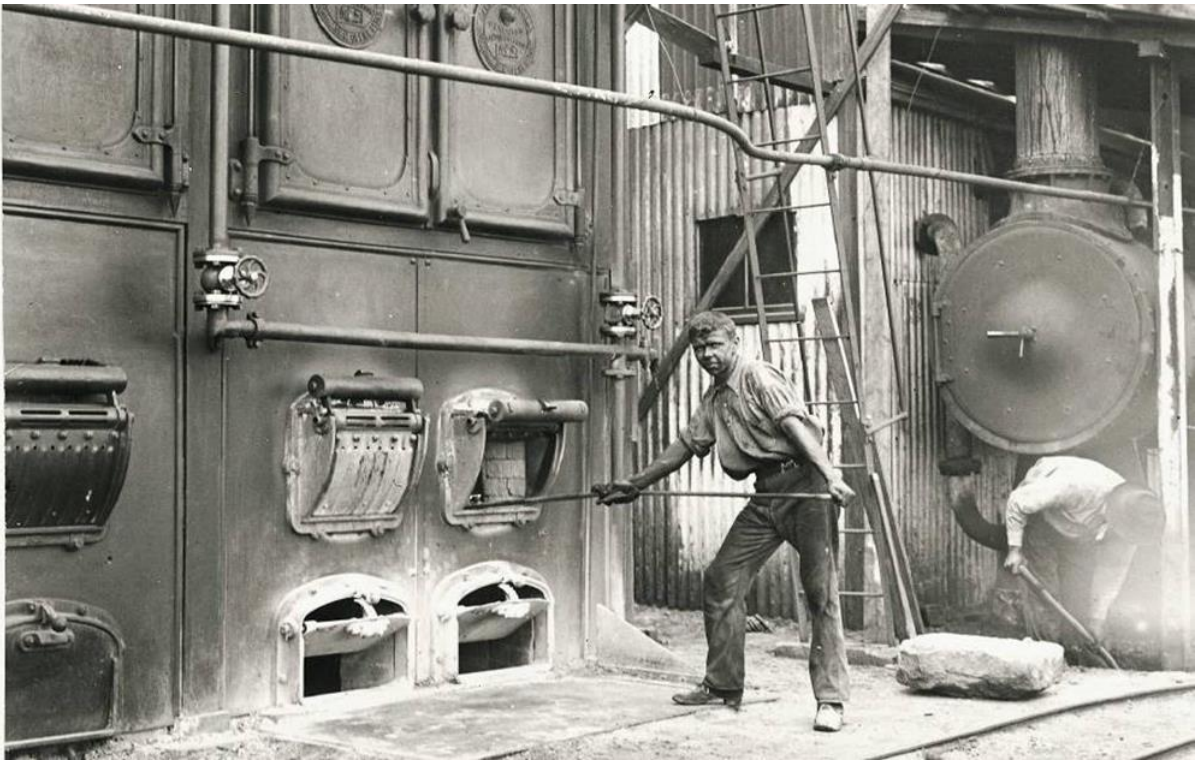
Plate 26: Worker using boiler at the established Mt Kembla Mine (Source: Arthur Wigram Allen)
