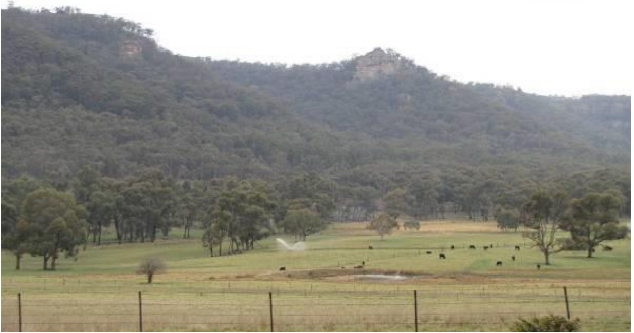
Photo 1: View from Springvale Road to the north-east showing rolling rises adjacent to alluvial areas in the foreground, and a convex talus slope rising to a vertical pagoda at the top of a short sandstone cliff section of the Angus Place HGL in the background (Photo: DECCW/Neville Pavan).
