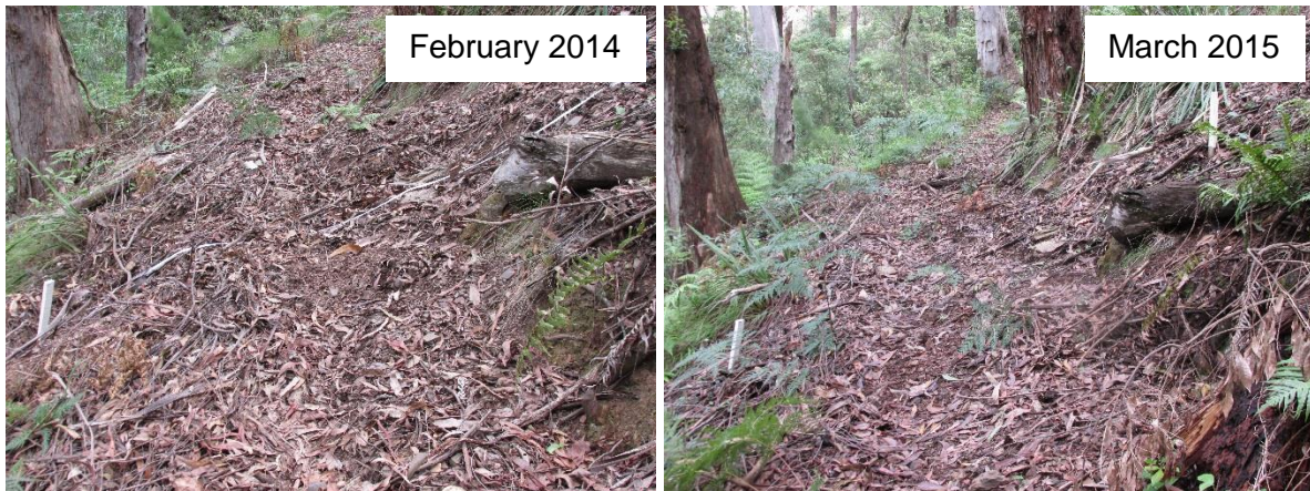
Figure 25: Photo points showing threshold trigger for track depth at site MSB002 Measurements are taken across the track, between two white pegs. February 2014 shows baseline track condition and March 2015 is when the trigger was detected.
