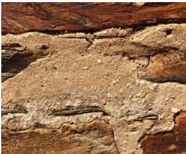
Figure 60: Flushed up pointing.
