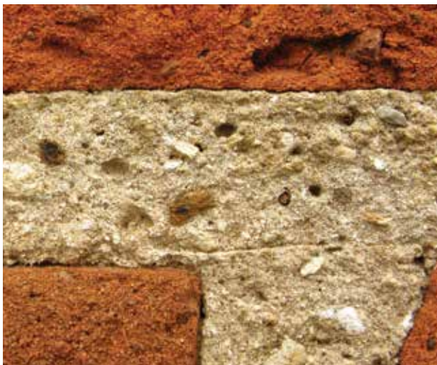
Figure 40: Internal view after abrasion.
