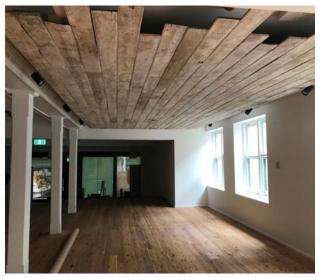
In this building in The Rocks, that contains remnants of a building from 1838, renovations revealed a timber ceiling from the late 1800s that had been over sheeted. The timber was removed and reinstated as an interpretive feature below a fire rated ceiling that protects remnants of an earlier lath and plaster ceiling.
