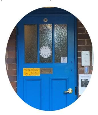
The door swing on this heritage door was altered to outwards and new complying exit handle installed. The original locks were deactivated and retained in place.
