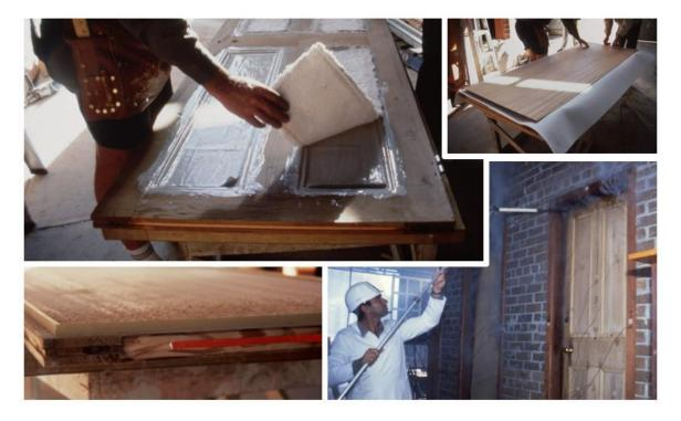
Timber panelled doors can be upgraded on their inside face to improve their fire resistance without affecting their external (i.e. corridor side) appearance, see <u>Upgrading the fire resistance of timber panelled doors</u>.
