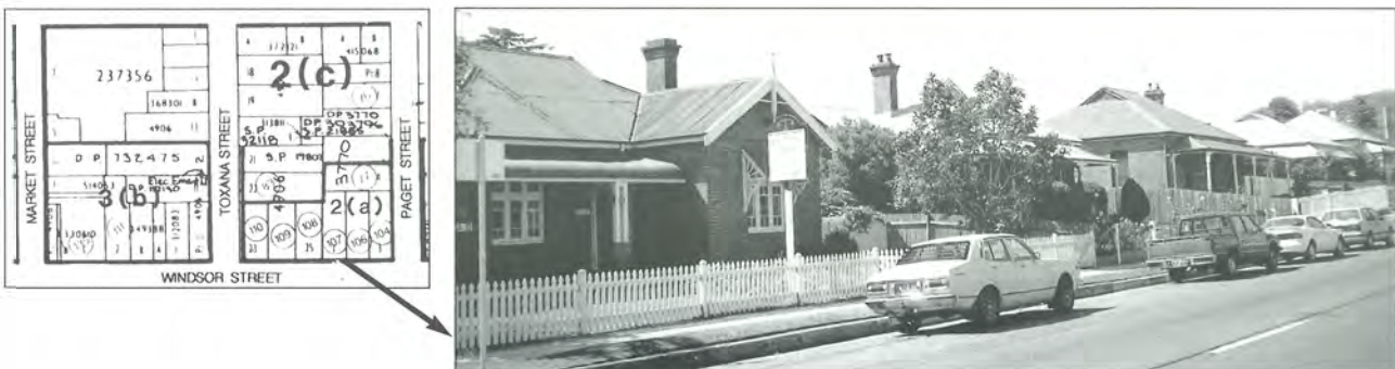
Figure 9 These old vernacular buildings in Windsor Street, Richmond derive much of their heritage significance from constituting an intact group, or precinct. A composite curtilage would follow the perimeter of the whole group of cottages, as shown on the map. Photo: Warwick Mayne-Wilson.
