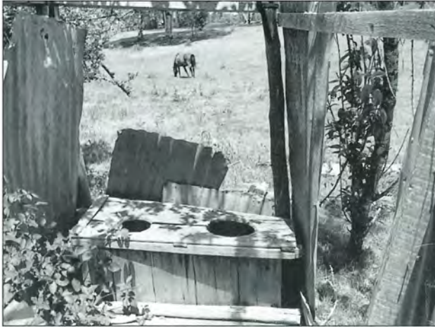
Figure 31 This old privy in the backyard of a miner's cottage in the Hill End conservation area is a significant feature that tells not only about sanitary arrangements in this gold mining town but also about family size and social behaviour. Its position at the back of the yard helps to define the curtilage for the rear of the property. Photo: David Beaver.
