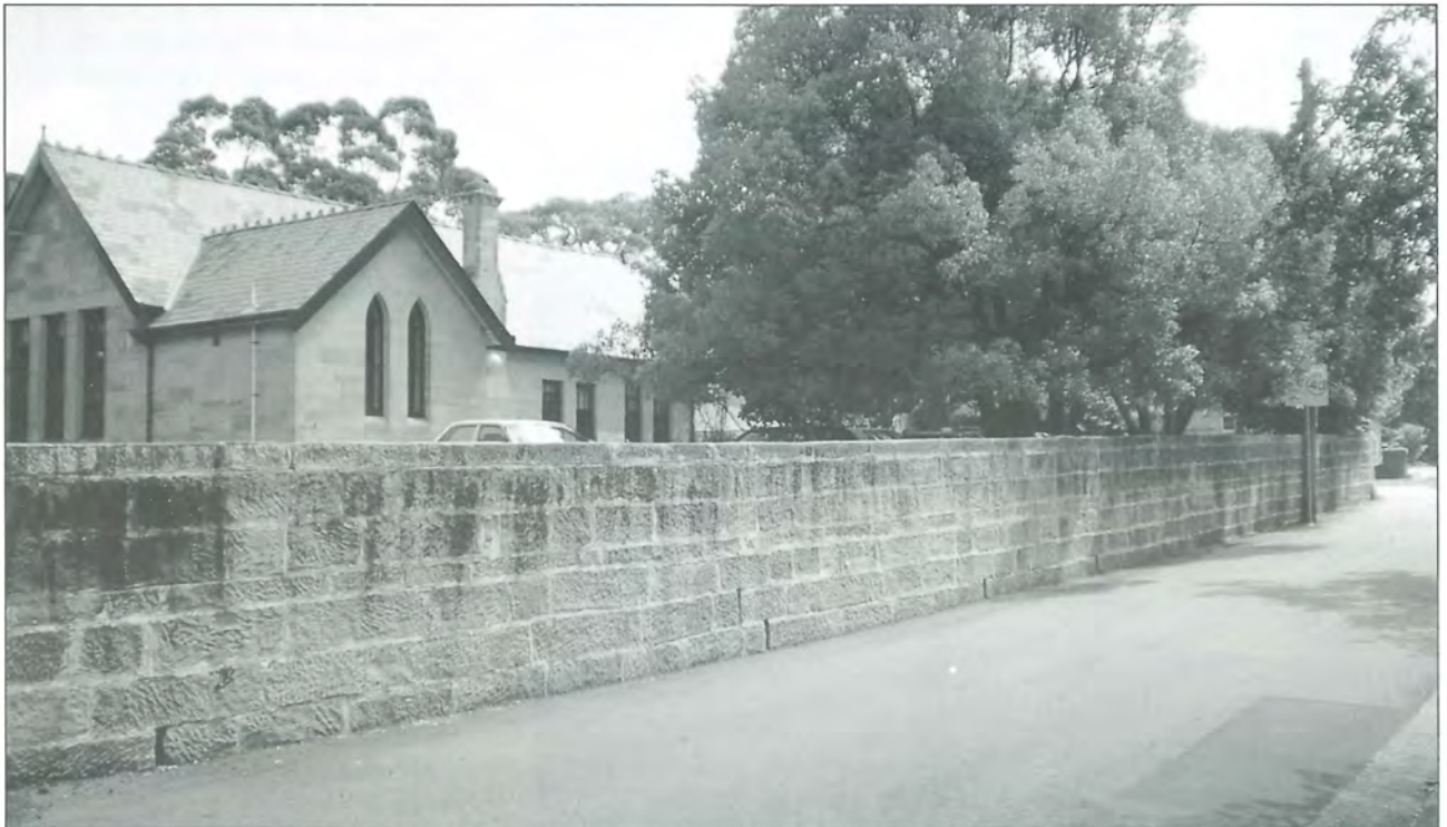
Figure 32 This original stone wall marks the boundary of the first sub-division in Stanley Road, Hunters Hill and is a significant heritage item because it clearly reveals part of the settlement pattern of the area. It could also be used to help define part of the curtilages for historic items, such as churches, mansions and schools, which were built within it. Photo: Warwick Mayne-Wilson.
