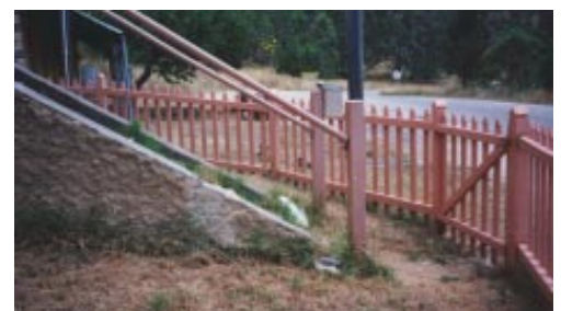
Ivy Cottage, front fence and garden Source: OCP 2000
