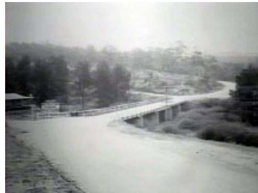
Lett River Bridge, State Highway 5 Source: ML, 1938
