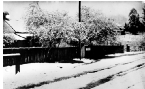
An undated view of the Post Office covered in snow Source: NPWS Hartley Image Collection
