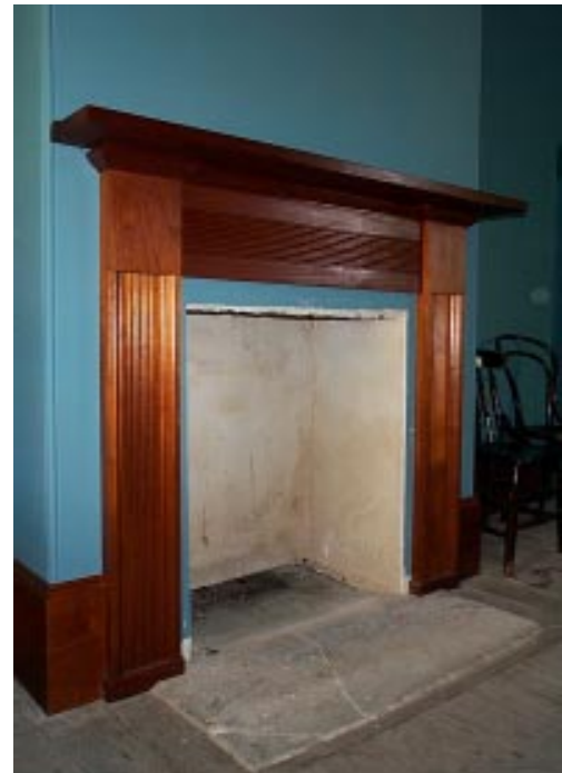
Detail of the fireplace Source: OCP Dec 2000
