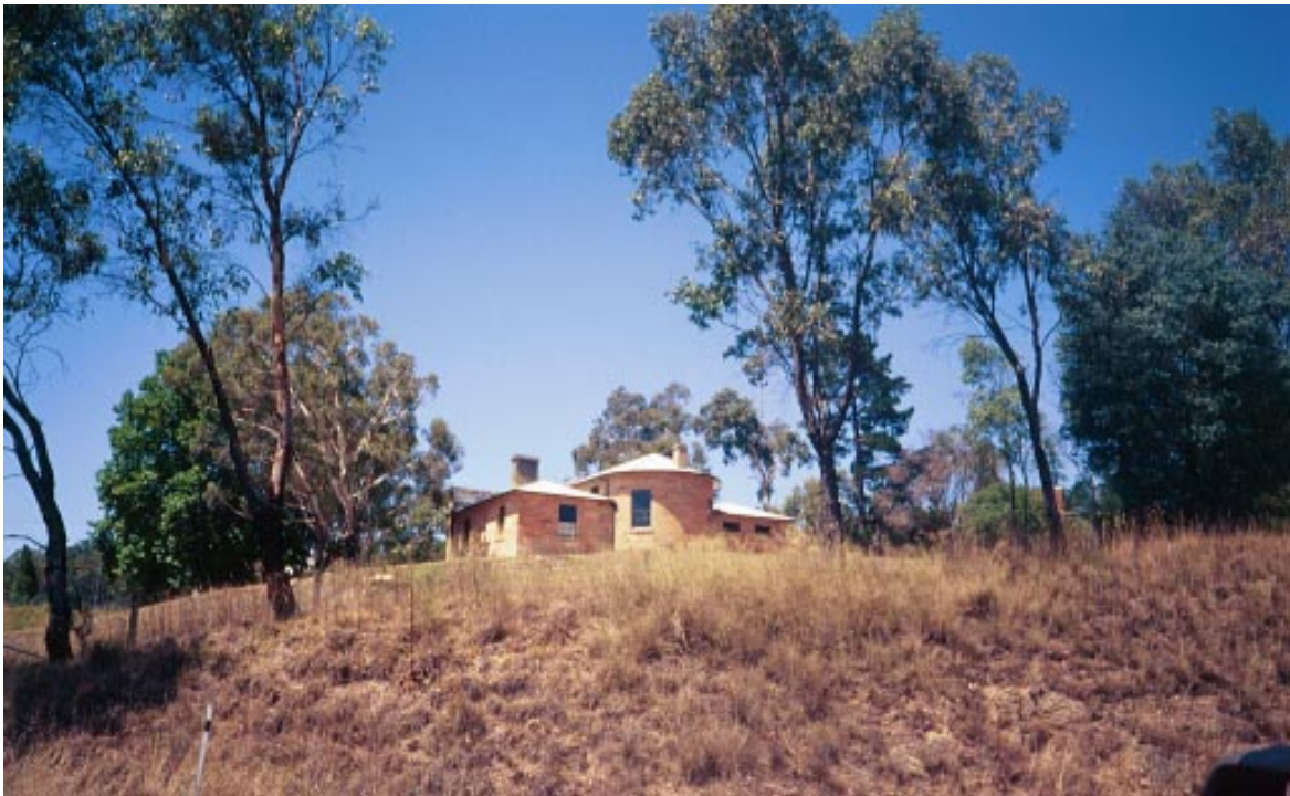
Current view of the rear of the Court House Source: OCP Jan 2001
