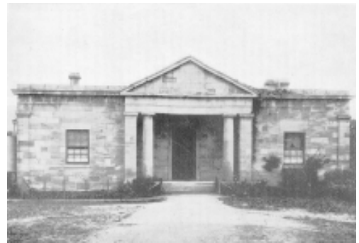
A view of the Hartley Courthouse in the late nineteenth century. The lace curtains and front garden indicate that it is no longer functioning as a courthouse Source: Forster et al, 1937
