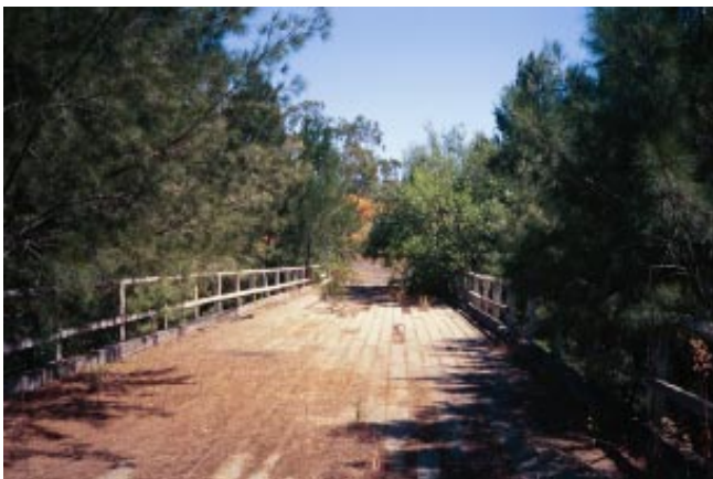
Current view of the River Lett Bridge OCP Jan 2001
