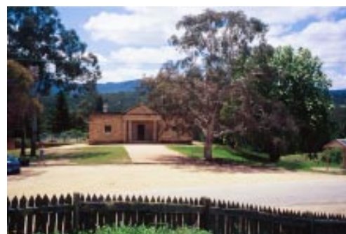
Current view of Hartley Courthouse and its forecourt OCP Jan 2001
