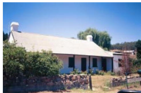
View of the remnants of the Post Office Garden Source: Gina Plate November 200
