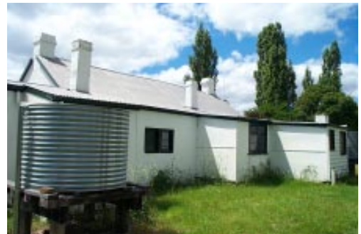
Current view of the additions to the rear of the former Post Office OCP Dec 2001
