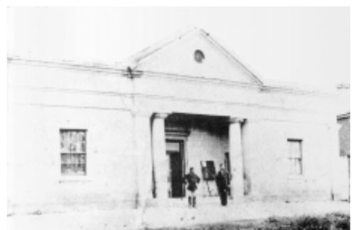
Mortimer Lewis' courthouses: Berrima, (top) and the three demolished courthouses: Bathurst, Newcastle, Yass
