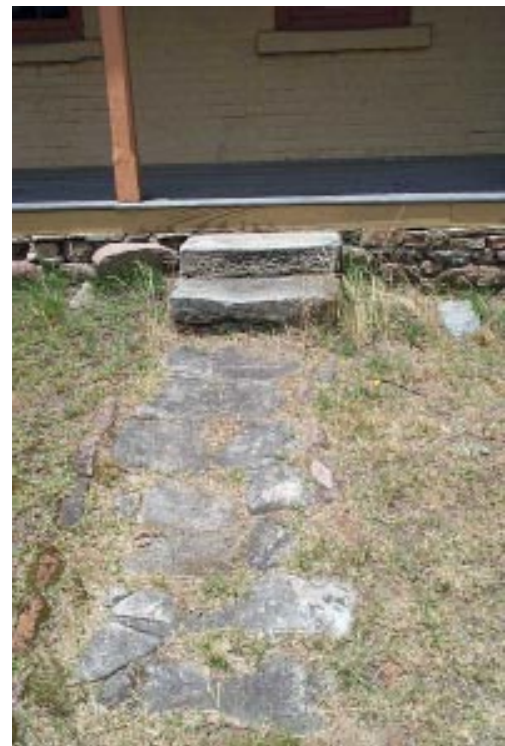
Old Trahlee original sandstone front path and steps Source: OCP 2001
