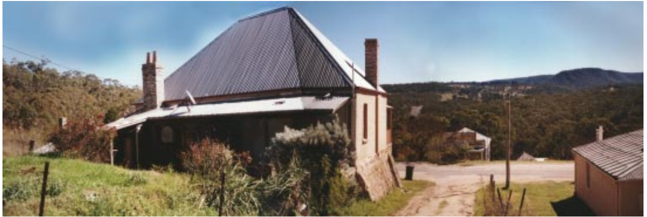
Rear garden of Ivy Cottage from lane Source: OCP 2001
