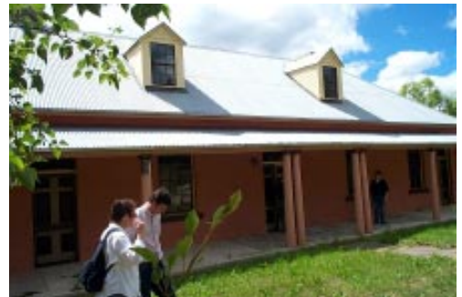
Current View of Royal Hotel Source: OCP Jan 2001
