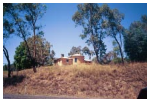
Current view of the rear of Hartley Courthouse OCP Jan 2001
