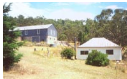
Current View of Corney's Cottage OCP Jan 2001
