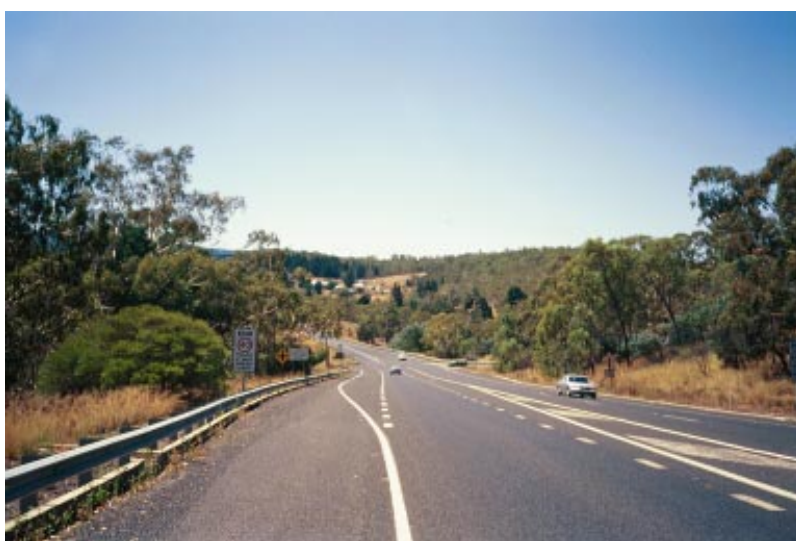
Current view of the village and turn off to Jenolan Caves heading east along the Great Western Highway Source: OCP Jan 2001
