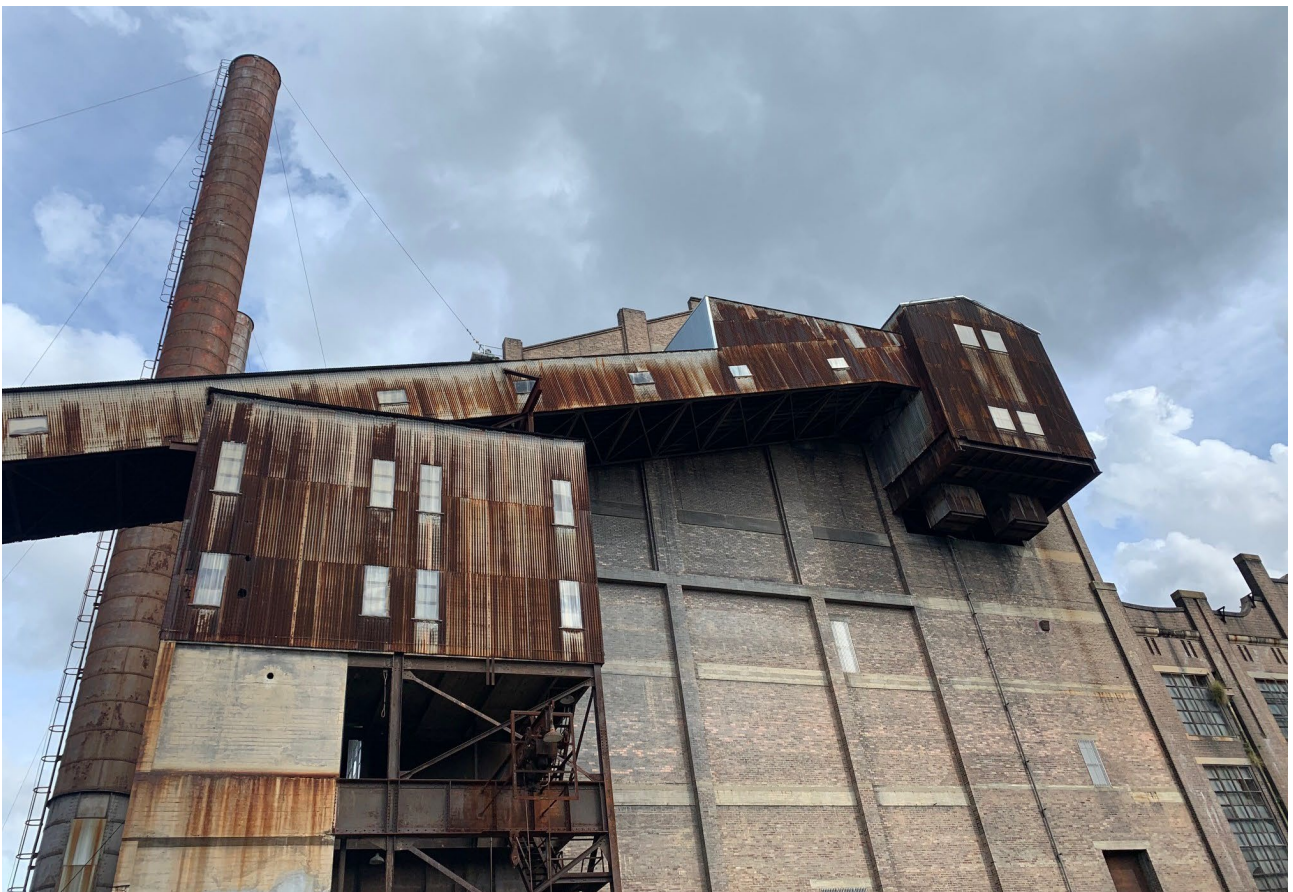
White Bay Power Station
