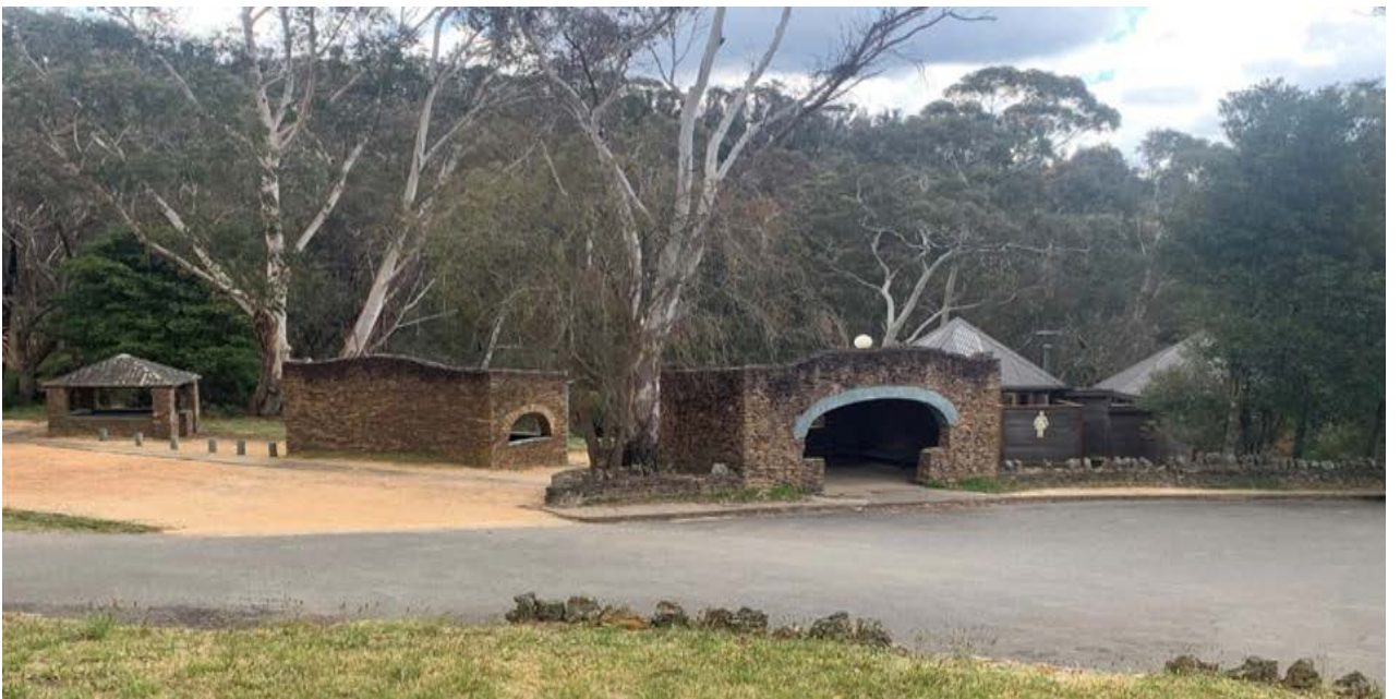
Figure 18 Picnic shelters, shelter and modern toilets adjacent to carpark
