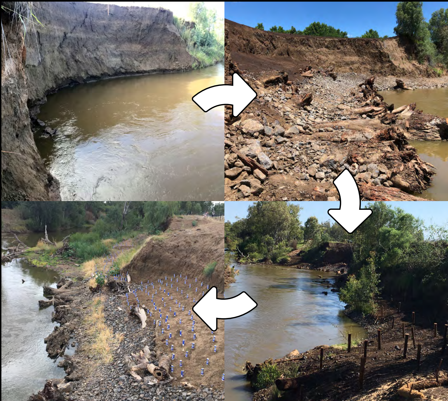
Figure 2 Rehabilitation of Gwydir River using installed wood and vegetation (photography: Peter Corlis, NSW Soil Conservation Service)
