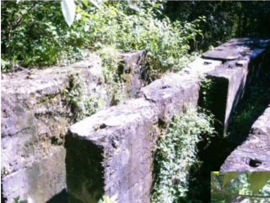
Figure 4-23: Winding engine foundations, Old Burwood Colliery site.
