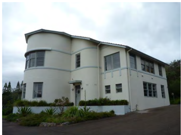
Figure 3.9 The primary (southern) elevation and eastern elevation of the Officers' Mess. The 1950s hipped roof has compromised its aesthetic significance. (Source: GML 2015)
