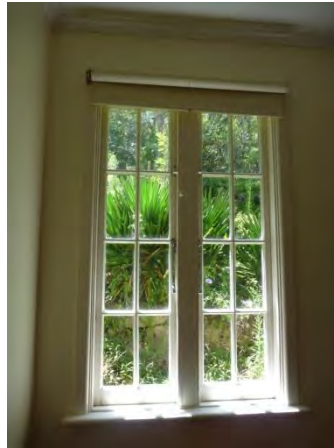
Figure 3.31 Early or original timber-framed casement window in the rear bedroom. (Source: GML 2015)
