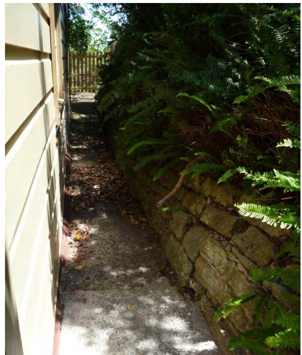
Figure 3.55 Sandstone block wall along the rear of the cottage. (Source: GML 2015)
