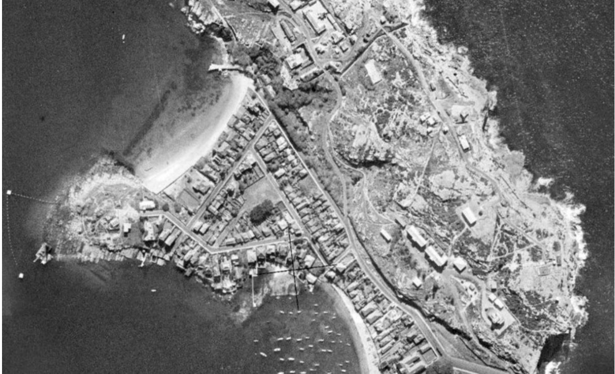
Figure 2.10 1943 aerial showing development at Green Point, Camp Cove and Gap Bluff .(Source: Department of Lands)
