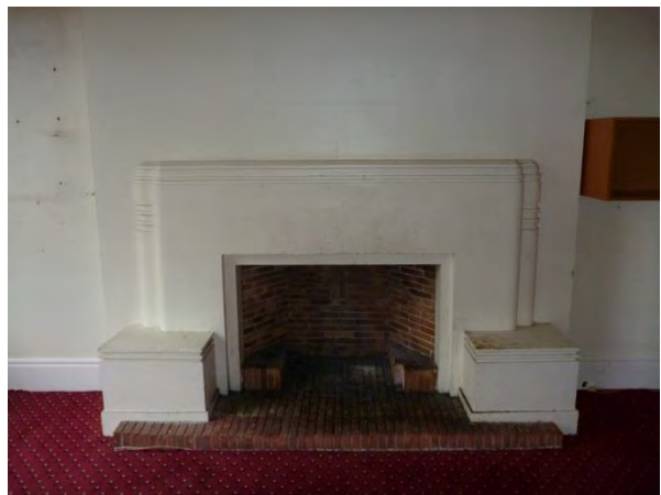
Figure 3.19 Original billiard room brick fireplace and moulded plaster surrounds on the first floor. (Source: GML 2015)
