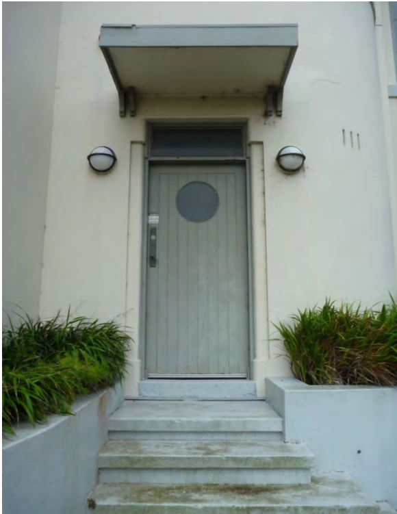
Figure 3.12 The original entrance, western elevation, with raised garden beds and concrete steps. The awning was constructed c1950s, replacing an earlier awning. (Source: GML 2015)
