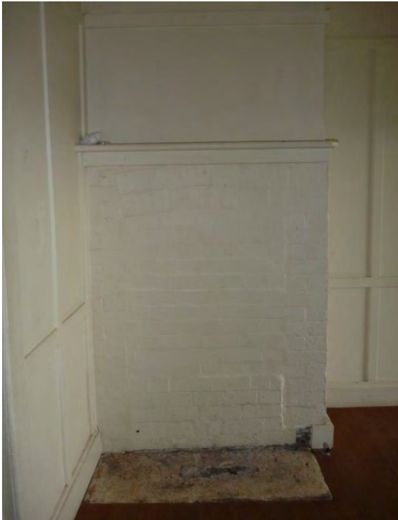
Figure 3.42 The original fireplace, mantelpiece and hearth in the western half of the cottage. (Source: GML 2015)
