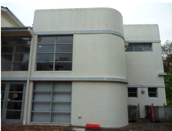
Figure 3.20 Eastern wall of the 1989 extension to the Officers Mess. (Source: GML 2015)
