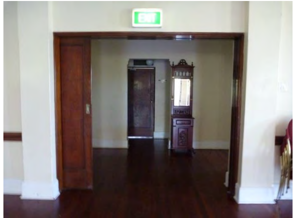
Figure 3.13 Original timber sliding doors from the ante room to the reception hall. (Source: GML 2015)
