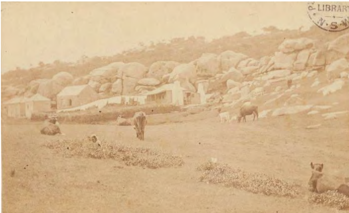
Figure 2.4 1869–1874 photograph of the Water Police Station and the associated timber accommodation buildings at Camp Cove. (Source: SLNSW SPF 808 a089808r)
