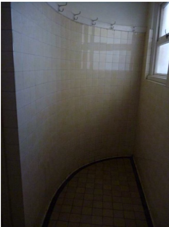
Figure 3.14 Original tiles and coat hooks within the ground-floor bathroom. (Source: GML 2015)
