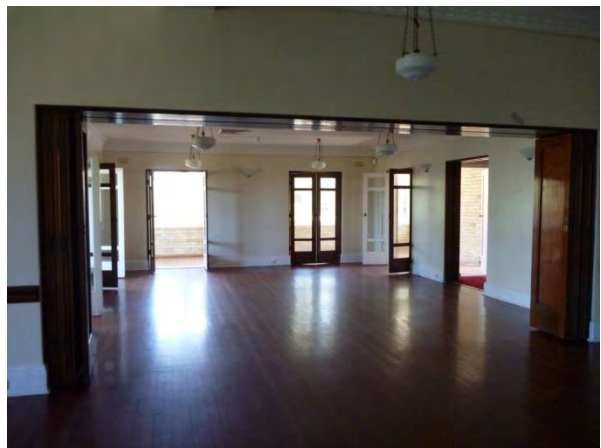
Figure 3.11 Interior view on the ground floor, looking west towards the mess room. The timber folding doors are original. (Source: GML 2015)
