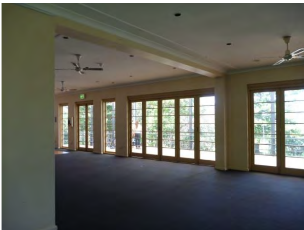
Figure 3.25 View of the highly modified interiors, showing the c1989 French doors and suspended ceiling. (Source: GML 2015)
