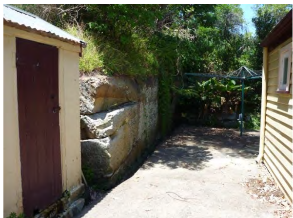
Figure 3.41 The original toilet block on the left, built into a cutting in the sandstone. The service wing is on the right. (Source: GML 2015)
