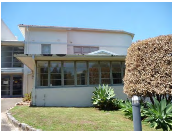
Figure 3.8 The western elevation of the Officers' Mess, showing the 1989 addition on the left. (Source: GML 2015)
