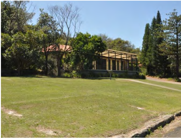
Figure 3.23 The Armoury, showing the c1989 verandah on the southern facade of the original building. (Source: GML 2015)
