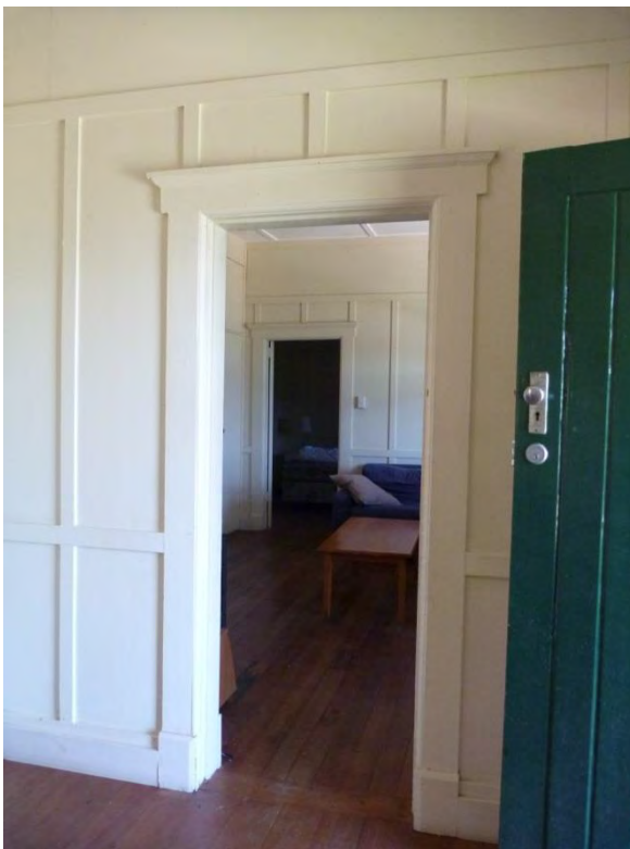
Figure 3.44 View from the dining room to the living room, showing the entablature architraves around a post-1952 doorway and an original doorway in the background. (Source: GML 2015)
