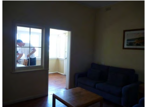
Figure 3.53 The original interiors of the cottage have been replaced. (Source: GML 2015)
