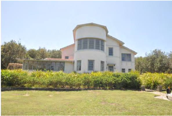
Figure 3.6 The primary (southern) elevation of the Officers' Mess. (Source: GML 2015)
