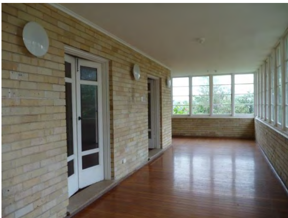
Figure 3.10 View of the enclosed verandah on the western side of the Officers' Mess, showing the early/original timber-boarded floor, blond brick walls and timber-framed French doors and casement windows. (Source: GML 2015)
