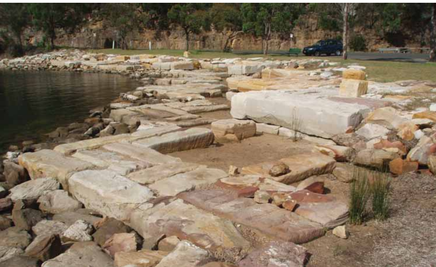
Figure 30: A seawall created at Bobbin Head, Cowan Creek, Hawkesbury River estuary, which highlights a number of the design principles discussed, including gentle slopes and a variety of habitats.
