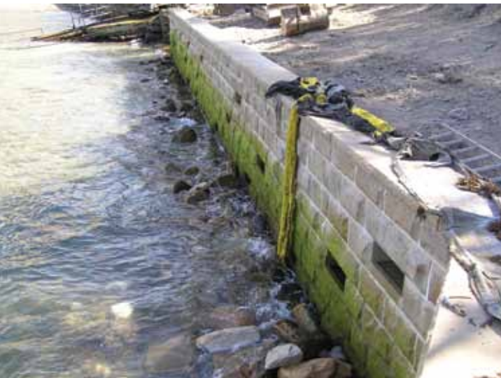
Figure 24: A seawall at McMahon's Point, Sydney Harbour, purposely designed to include pools in the structure for habitat, and boulders at the toe for additional habitat.
