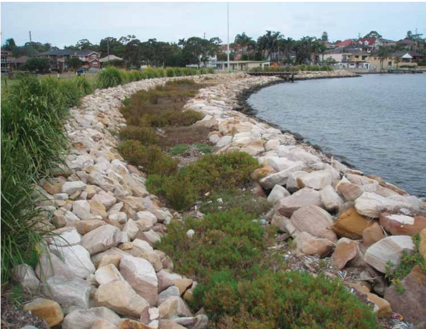
Figure 20: Before (right) and after (below) shots of the seawall at Kogarah Bay, Georges River, showing a step-type seawall with a bench of saltmarsh vegetation.
