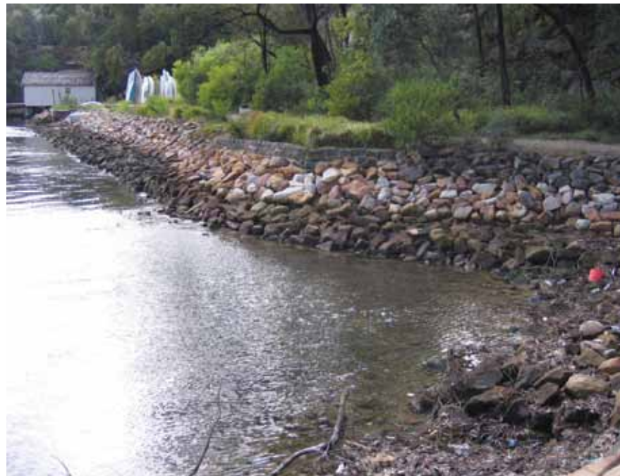
Figure 13: Before (above) and after (right) shots of seawall habitat improvement works at Quakers Hat Bay, Sydney Harbour, showing how the boulders were used to increase total habitat surface area and complexity to a traditional vertical stone block seawall.
