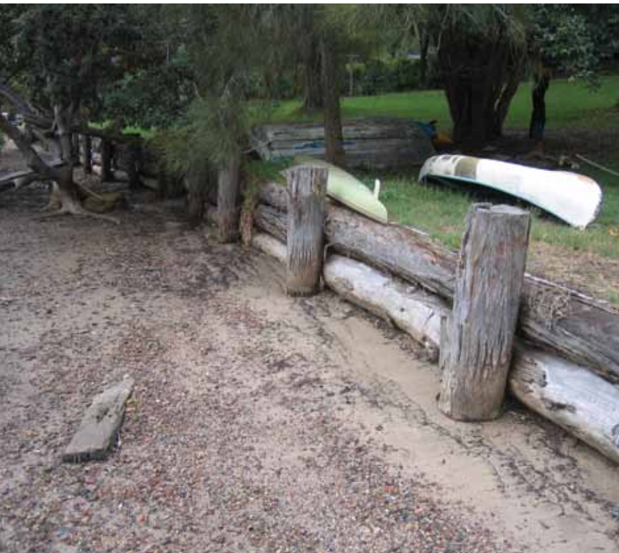
Figure 28: Example of a seawall made out of logs, Elvina Bay, Pittwater (left).
