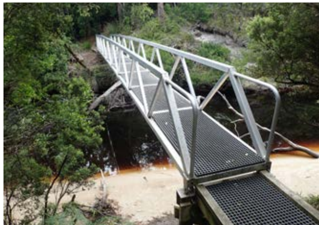
Photo: Example fixed bridge, Milford Creek, Tasmania
