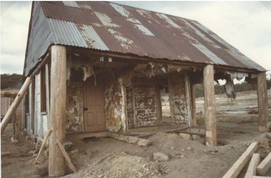
Campbell House during the restoration works. This is the southern end of the building. Source: NPWS Hurstville (now DECC)
