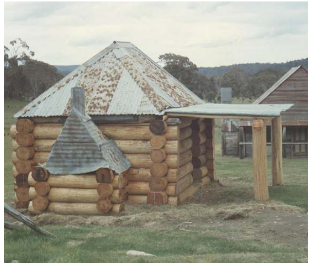
The completed Cheese Hut Source: NPWS Tumut
