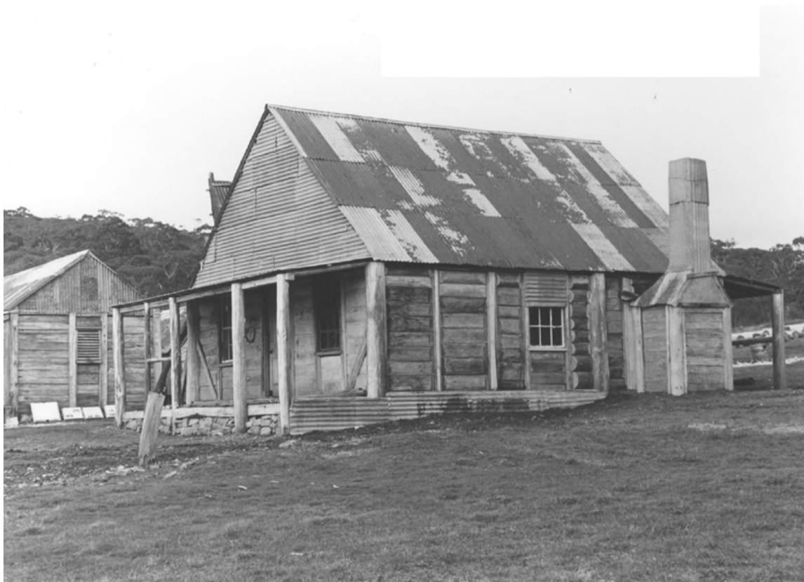
Campbell House after the restoration works. Note that the side door is now a window and that the house has been raised. Source: Phyllis Dowling Collection
