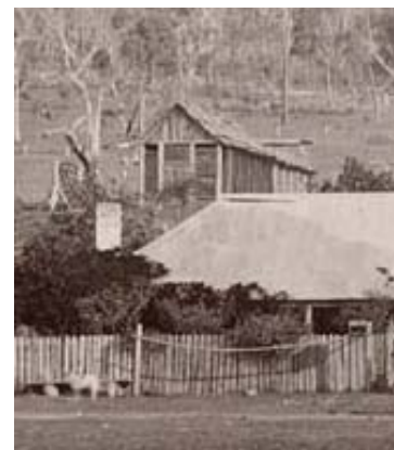
Detail of the Lampe's slab barn
