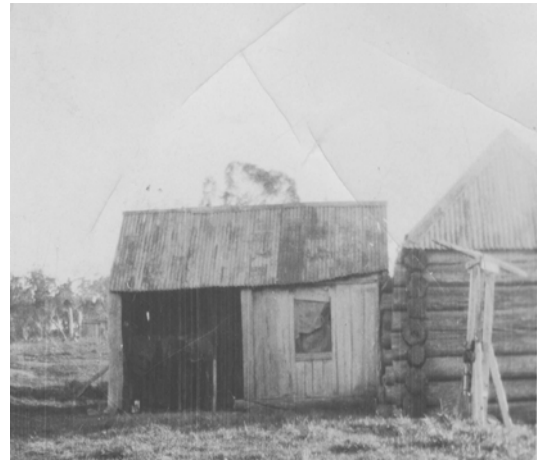
Detail of the de Salis hut circa 1937 showing the slabs
