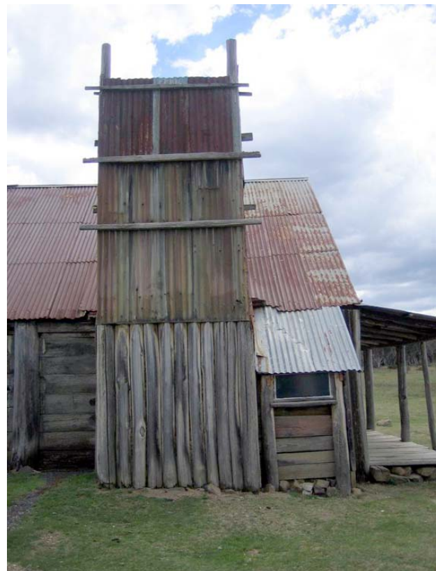
Recent view of the chimney to the Campbell House. Source: OC+P
