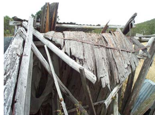
Remnants of the bark roof of the slab hut, Yanunbeyan National Park
