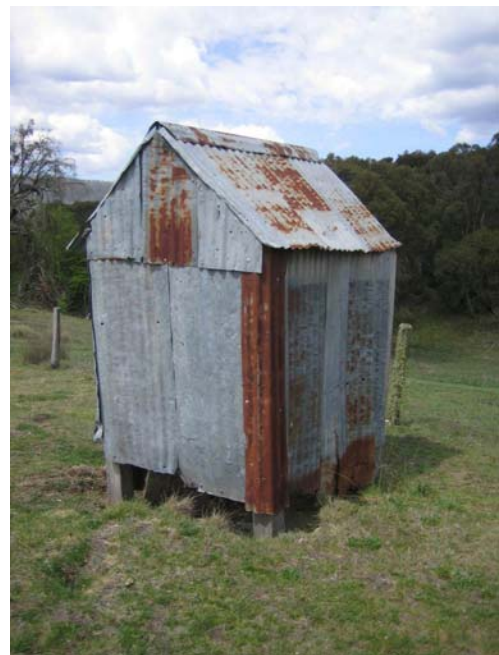
The larger outhouse, 2006 Source: OC+P
