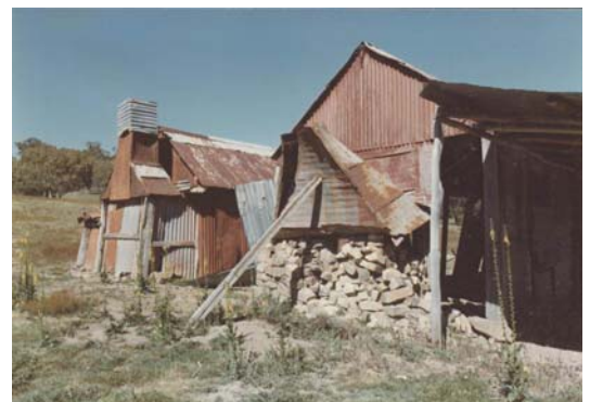
View of the Southwell House in 1982 before works commenced
