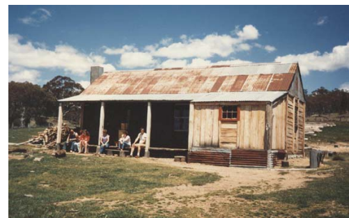
Szwed House after the restoration works. Source: Phyllis Dowling Collection
