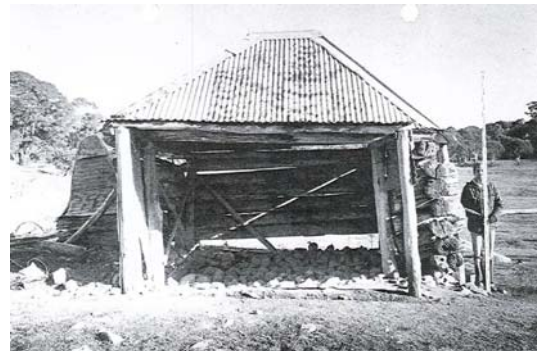
Photogrammetric recording of the Cheese Hut, 1981 Source: NPWS Hurstville (now DECC)
