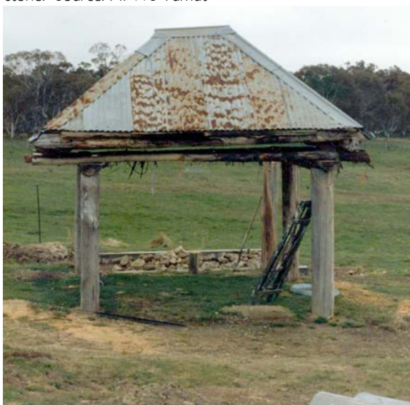
The Cheese Hut during the rebuilding, 1987. Note that the roof structure and the logs immediately below were retained in their entirety. Source: NPWS Tumut
