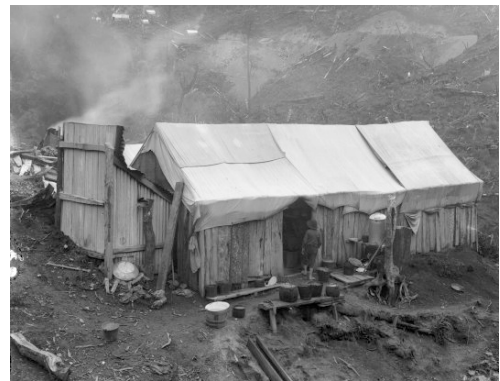
Slab but with a canvas roof in New Zealand
