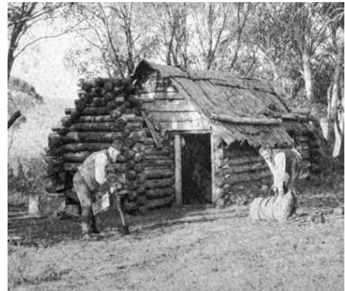
Rabbiters Log Cabin, with log chimney, Mt Wellington District, VIC. Note the similarity of the base of the chimney to the Cheese House Source: Museum of Victoria
