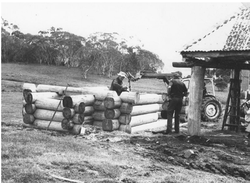
The Cheese Hut during the rebuilding, 1987. Note that the roof structure and the logs immediately below were retained in their entirety. Source: NPWS Tumut
