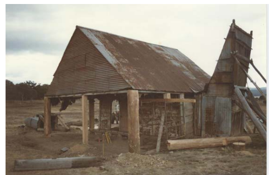
Campbell House during the restoration works. Source: NPWS Hurstville (now DECC)
