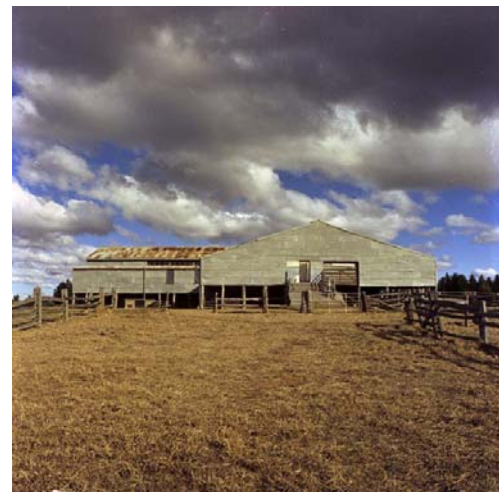
Recent view of the Yarralumla Woolshed Source: ACT Heritage Library 007101
