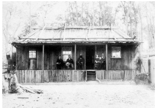
Slab hut at Bega with a bark roof held down by saplings Source: ML At Work and At Play still 02041
