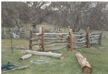
Repair works to the yards, 1987 Source: NPWS Hurstville (now DECC)
