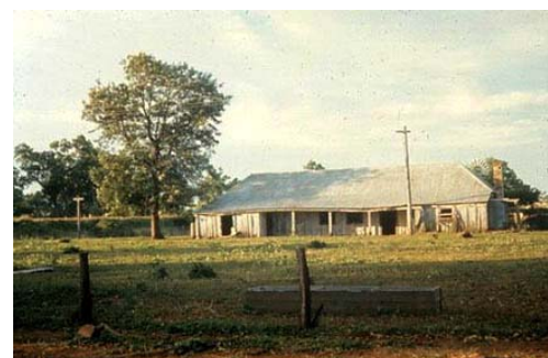
Dundullimal Homestead Source: Australian Heritage Photographic Library rt05897
