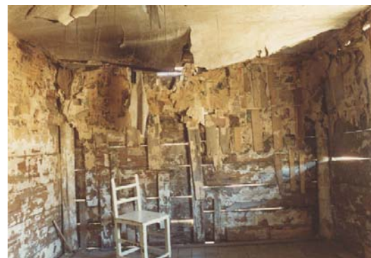
Remnant linings within the Campbell House Source: NPWS Hurstville(Now DECC)
