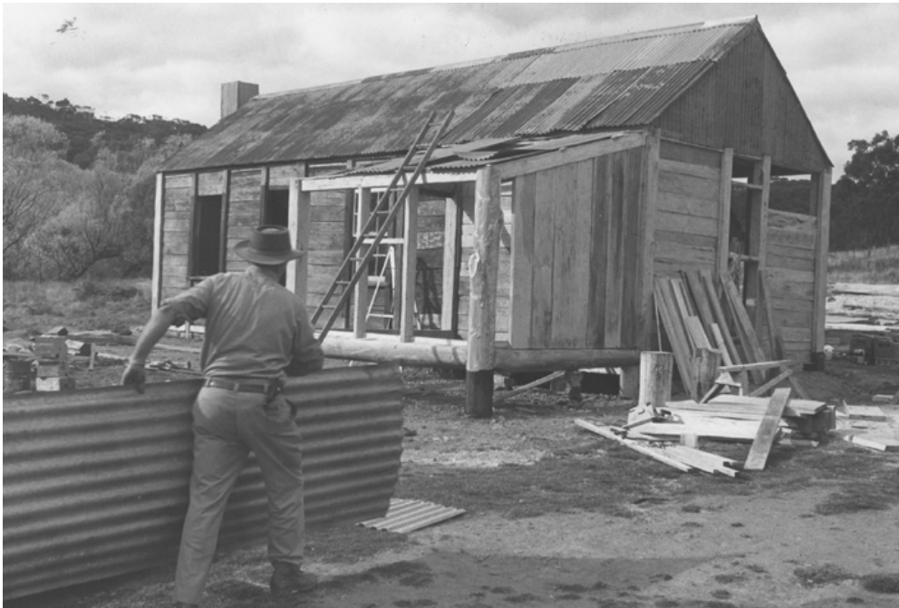
Szwed House during the restoration works. Source: Phyllis Dowling Collection
