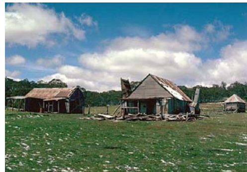
View of Coolamine taken by Max Bourke, 1978 Source: Australian Heritage Photographic Library
