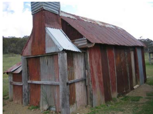
Recent view of the Kitchen Block Source: OC+P
