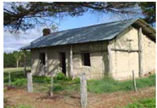
Pisé hut at Glenburn Source: Environment ACT
