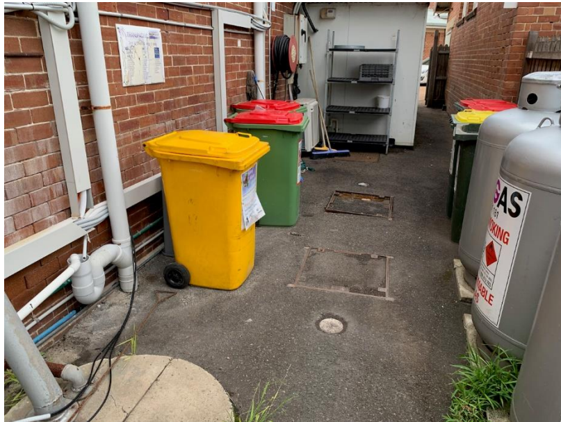
13 Waste bins behind the Boilerhouse.
