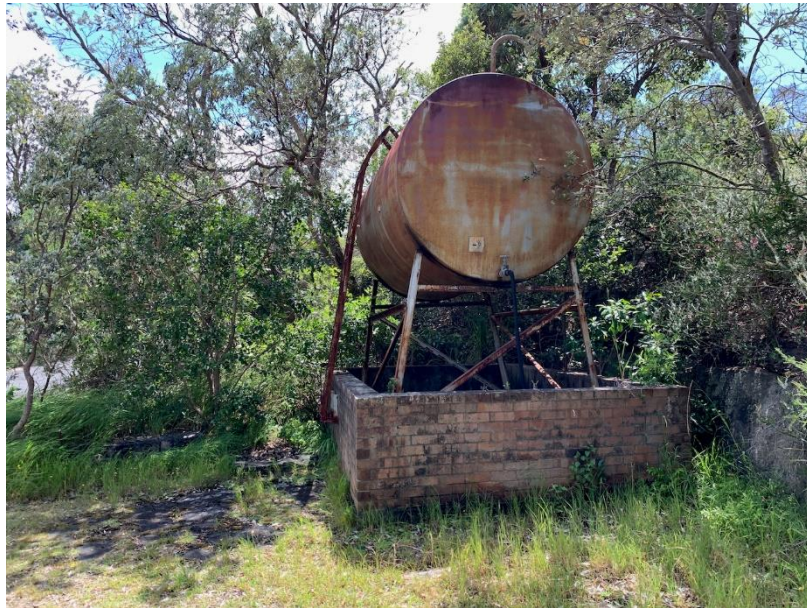
47 The Aboveground Storage Tank located opposite Building A18 Former Locomotion Shed.
