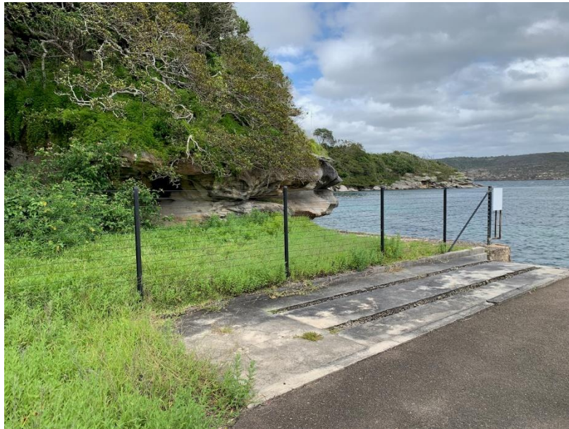
37 The fence installed near the southwest end of Building A14-17 to limit public access to Cannae Point (CoA 76).
