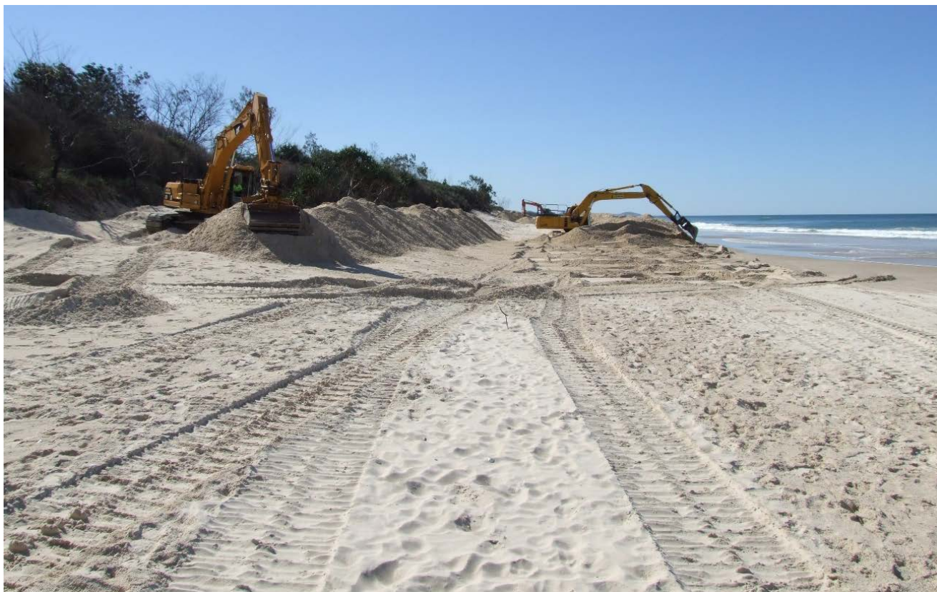
Figure B3.12 Beach scraping at New Brighton Beach, Byron Shire Council (Photo: B Fitzgibbon/Byron Shire Council)
