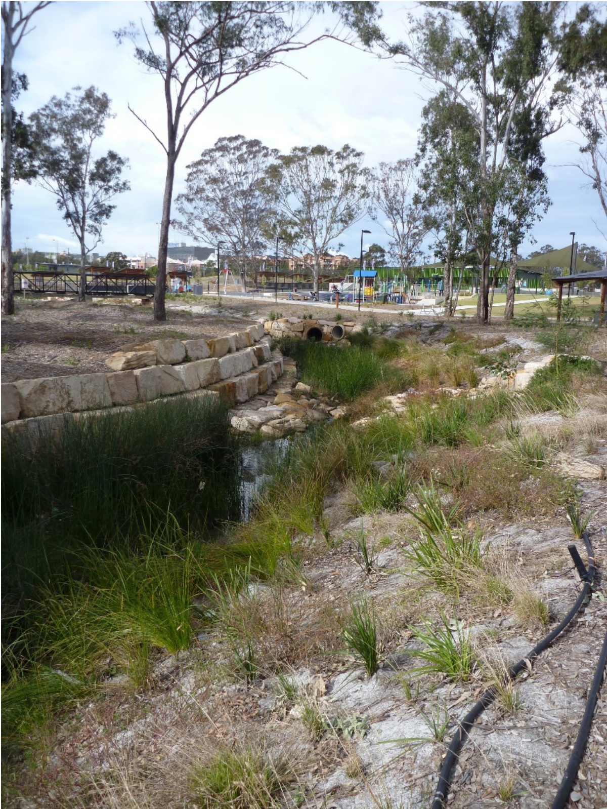
Figure B3.19 An example of water sensitive urban design: vegetated swale with floodway, Bankstown (Photo: P Vella/OEH)
