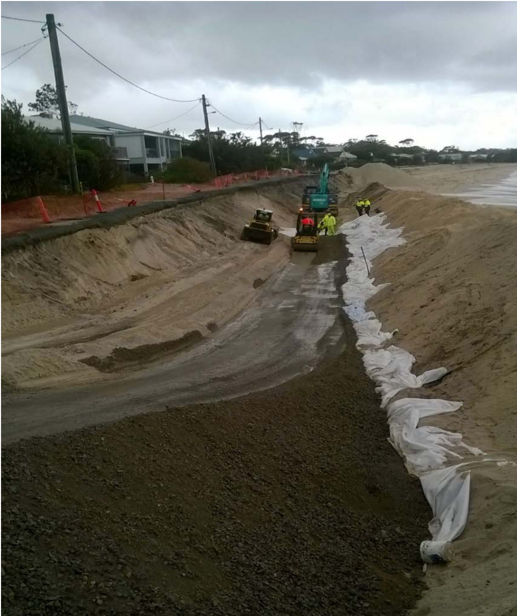
Figure B3.11 Beach nourishment, Jimmy's Beach (Photo: Great Lakes Council)
