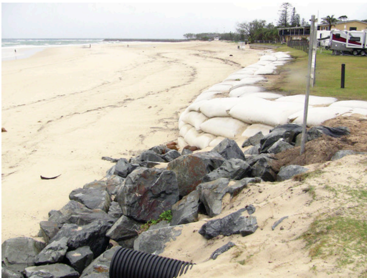
Figure B3.10 Coastal protection works, Kingscliff (Photo: P Davies/OEH)
