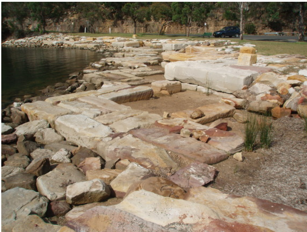
Figure B3.18 Environmentally friendly seawall made with sandstone blocks at Bobbin Head, Cowan Creek, Hawkesbury River estuary (Photo: D Wiecek/OEH)
