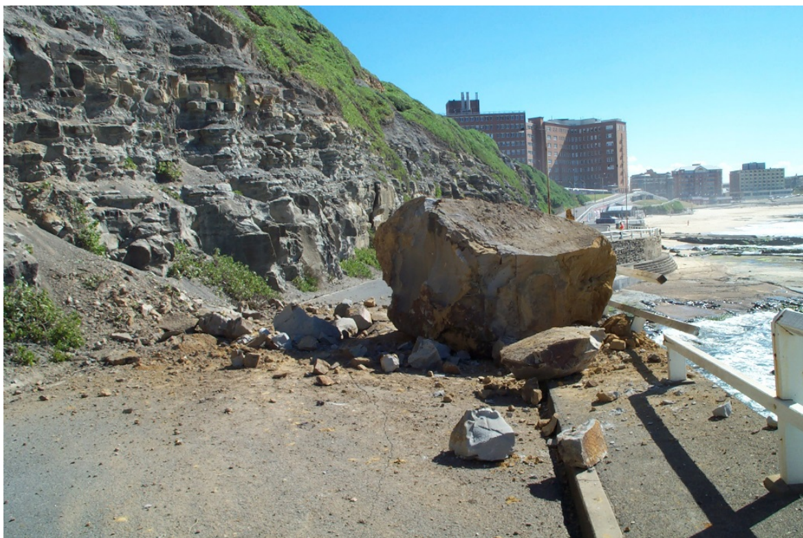
Figure B2.17 Rockfall from coastal cliff, Newcastle, October 2002 (Photo: OEH)
