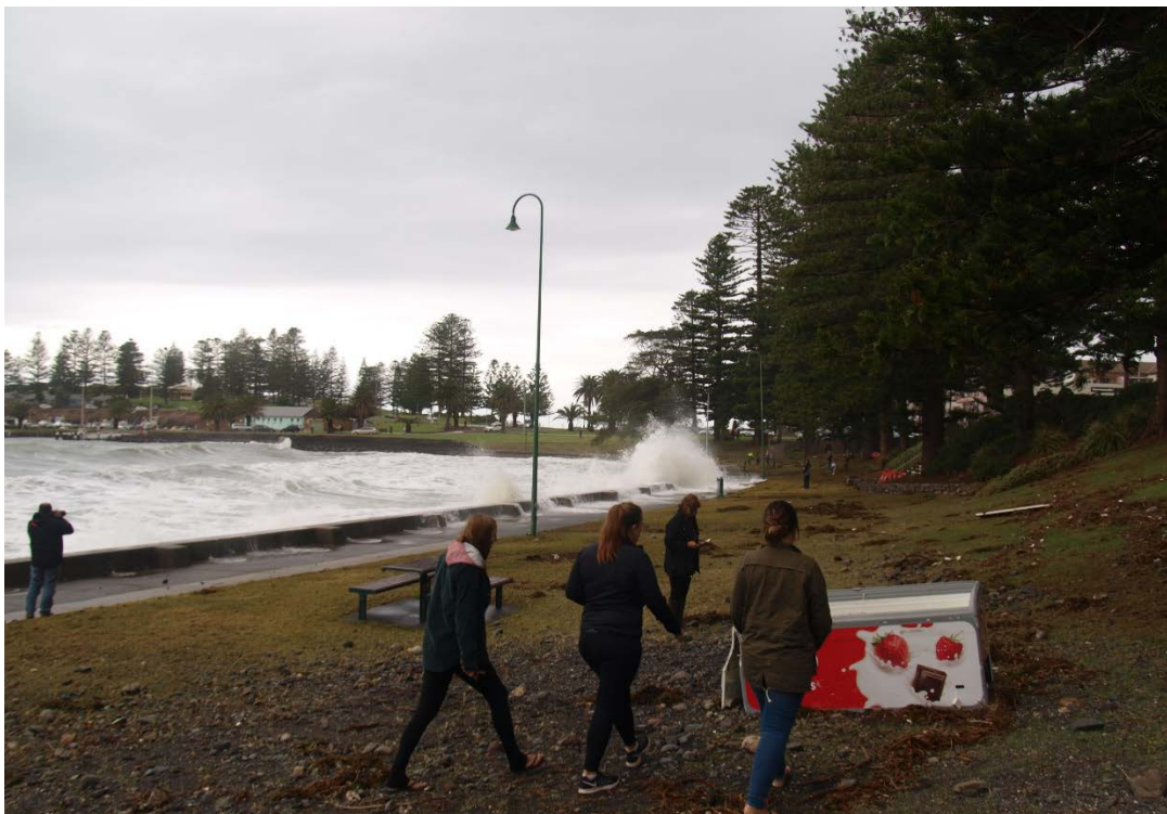
Figure B2.15 Waves overtopping seawall at Kiama Harbour depositing debris on foreshore, June 2016 (Photo: D Wiecek/OEH)
