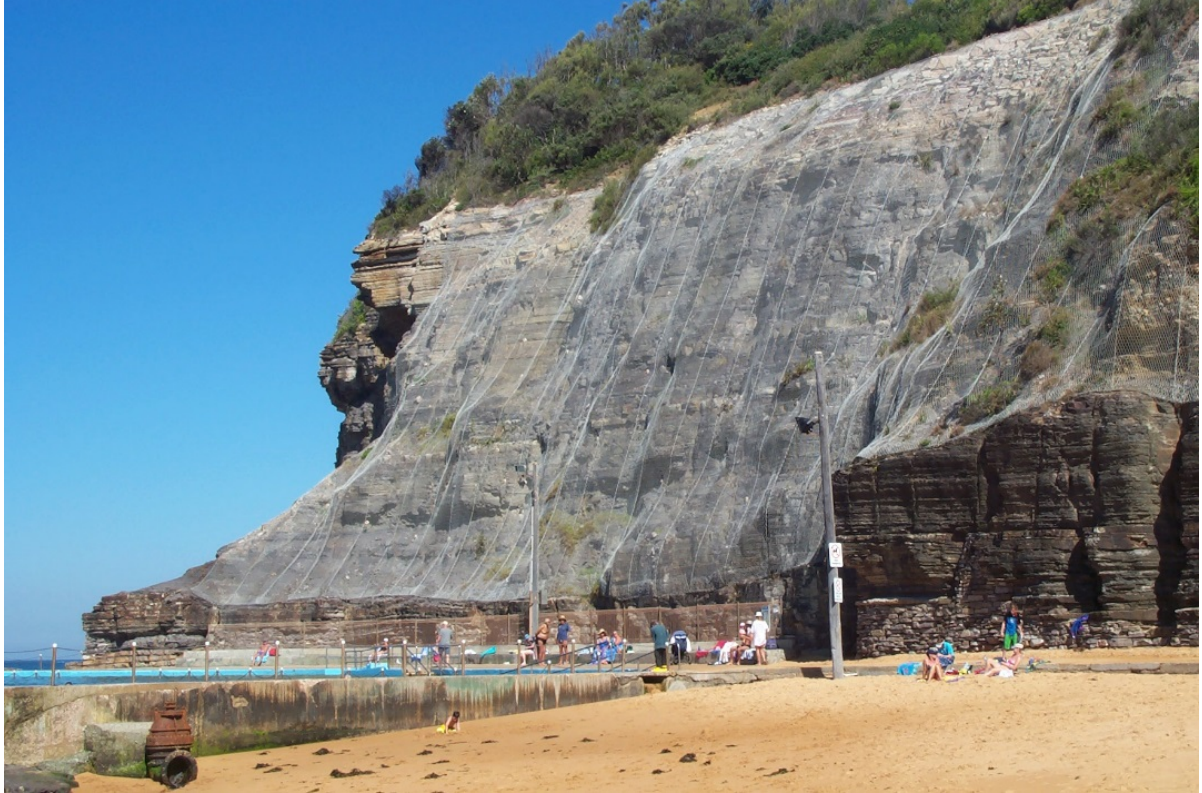
Figure B2.18 Cliff protection works, Bilgola beach (Photo: D Hanslow/OEH)
