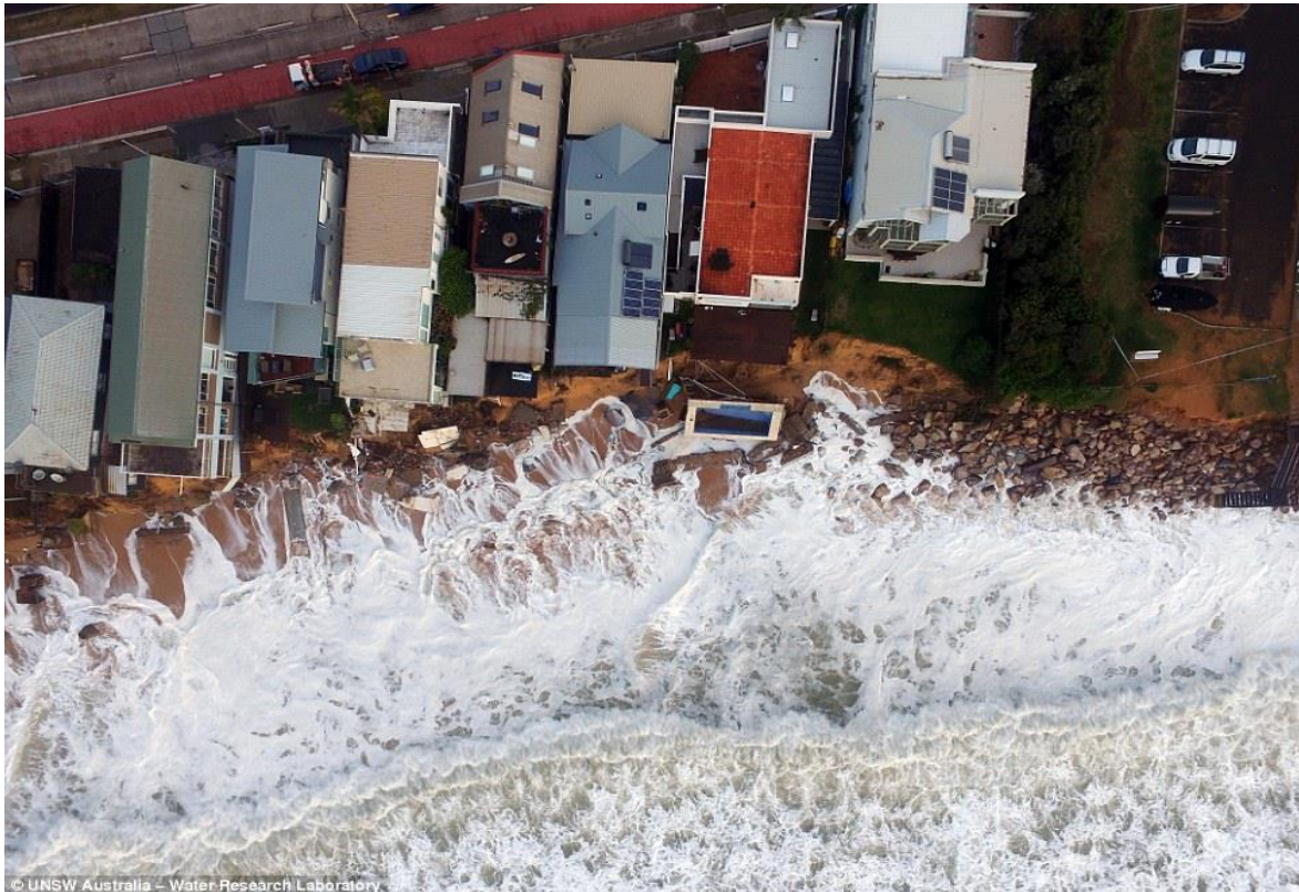
Figure A4 Erosion at Collaroy Beach, June 2016 (Photo: UNSW Water Resources Laboratory)
