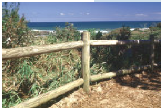
Figure 4.7d Post and rail fence, Angourie
