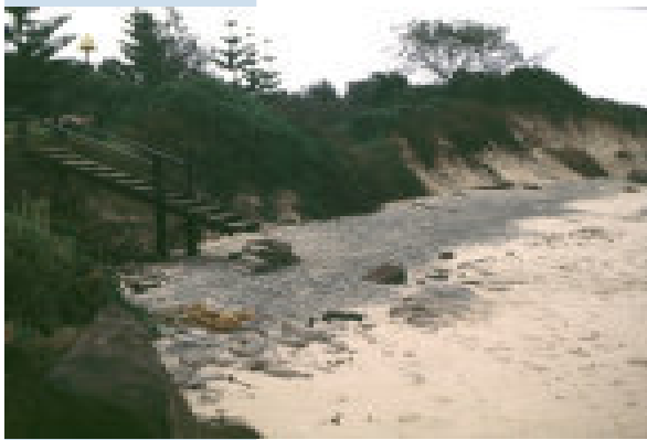
Figure 4.12b Seaward ends of stairways need to accommodate erosion.
