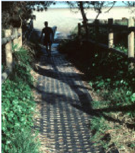
Figure 4.10c Recycled conveyor belt provides flexible, durable surface suitable for disabled access.
