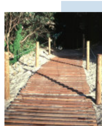
Figure 4.8 Pedestrian board and chain access. Note how the bounding fence is positioned close to the boards.
