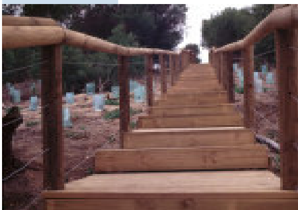
Figure 4.12c Staircase provides access across hind dune, protecting vegetation.
