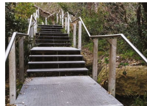
Figure 50 FRP stairs (Context, 2016)
