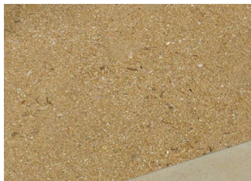
Figure 48 Cement stabilised decomposed granite path (Context, 2016)
