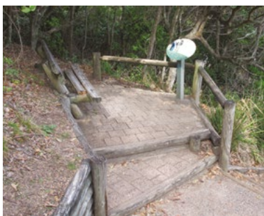
Figure 80 Existing circular signs to be removed (Context, 2016)
