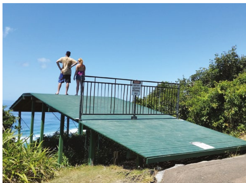
Figure 54 Existing hang glider launch ramp poses an ongoing safety issue (Context, 2016)
