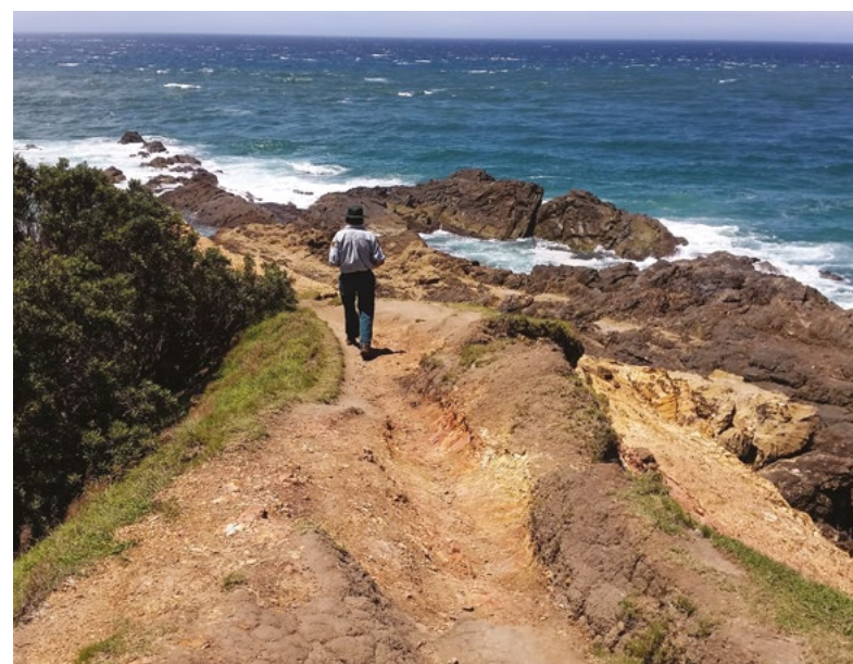
Figure 19 Erosion past the lookout at Little Wategos (Context, 2016)
