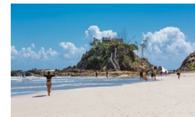
Figure 30 Fisherman’s Lookout is structurally unsafe and in need of immediate repair (Context, 2016)
