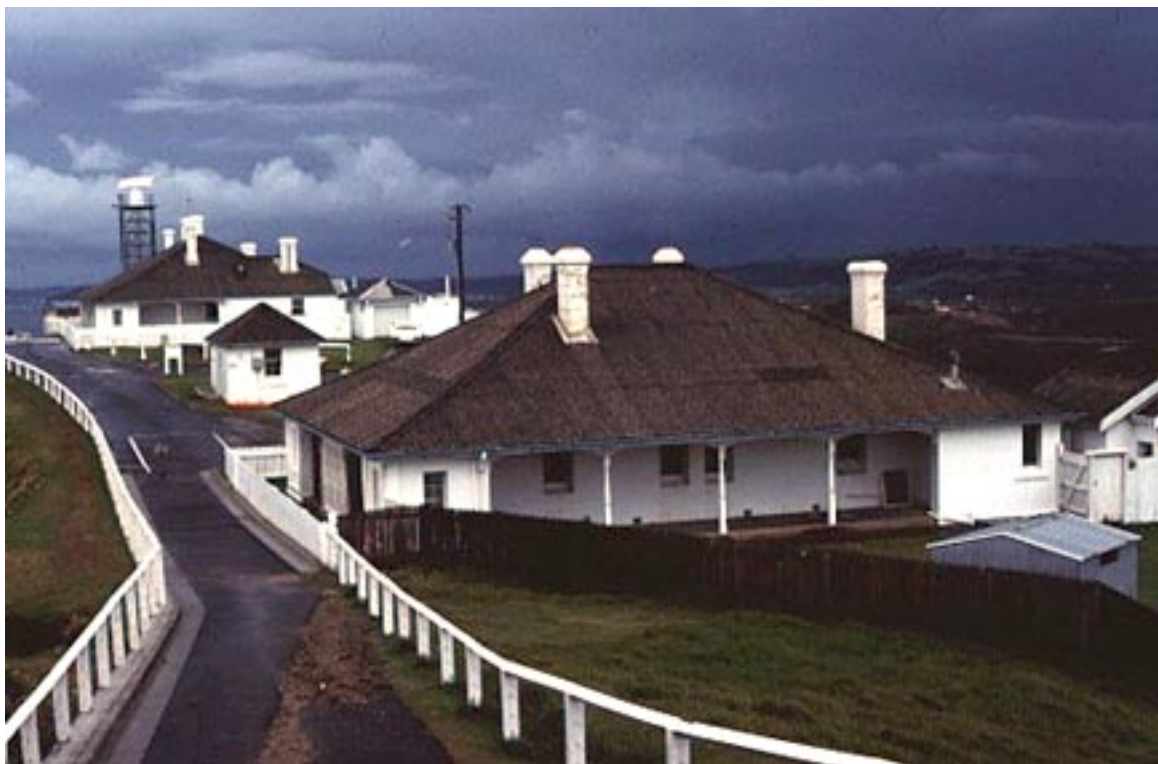
View of the quarters looking south in 1983 showing the radar tower on the south side of the former Assistant Lightkeepers' quarters. Source: DEW Image number rt05468
