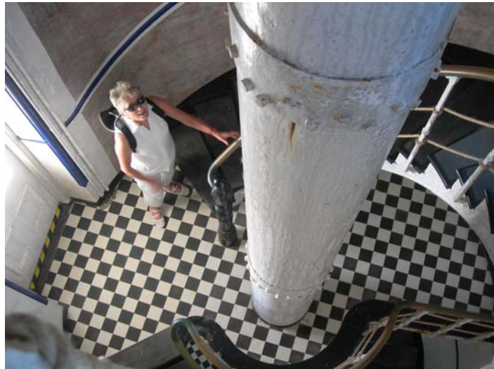
Figure 30: Inside the tower from above. Source: Ellsmore 2008.
