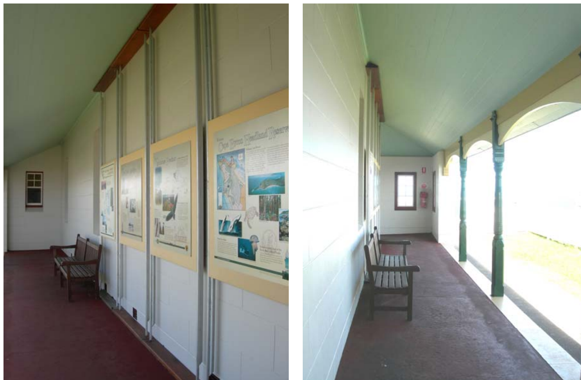
Views of the south verandah of the former Head Lightkeeper's quarters
