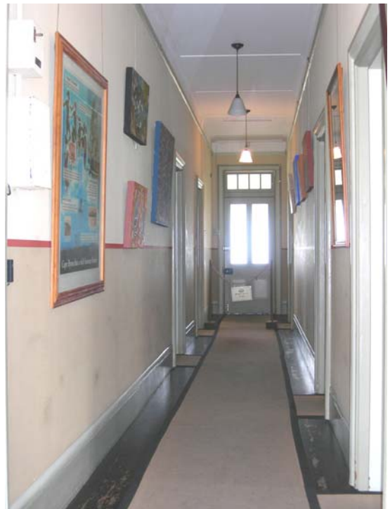
Plan of the quarters, and a view down the hallway from the front door. The uses of the rooms have changed since this plan was drawn and laundry has been partitioned to create a secure storeroom with separate corridor to the rear access door. Source: Pratten & Irving 1991 (left) and Ellsmore 2008 (right).
