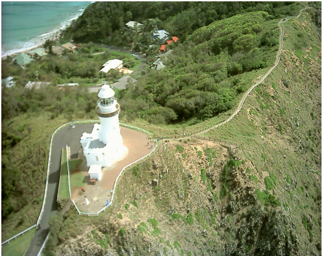
View of the Lighthouse and immediate surroundings from above from the south east
