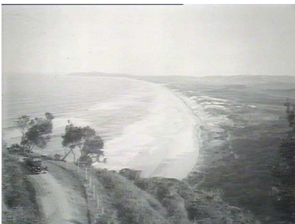
Figure 6: Car on road to Lightstation with Tallow Beach in background, circa 1920. Source State Records GPO1-24262.
