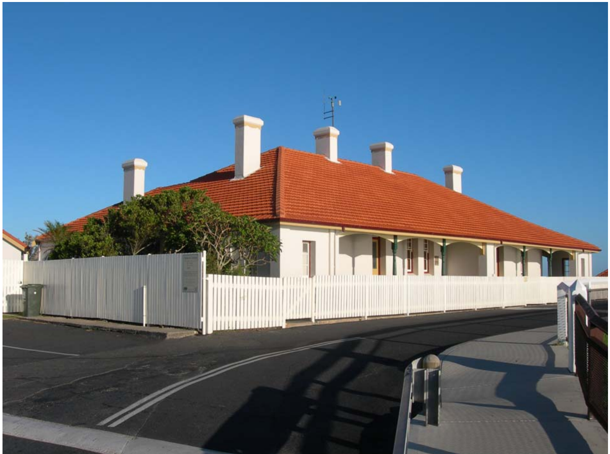
View of the former Assistant Lightkeepers' quarters.
