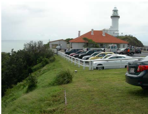
Views across the central precinct parking area taken from the south (left) and north (right). The embankment in the left view was created at the time of construction by dumping the builders' spoil into the former depression. The original fence line was parallel with the walls of the quarters.
