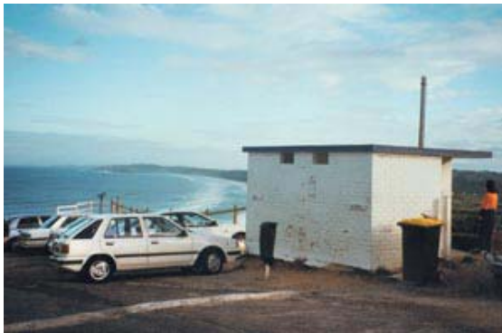
Figure 11: Toilet block at the precinct, circa 1980. Source: ncph036
