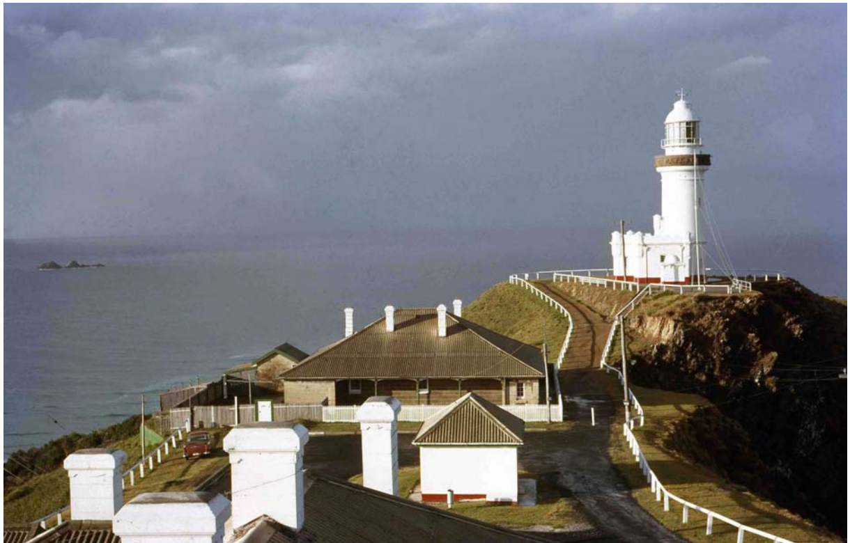
View of the northern portion of the lightstation showing the former Head Lightkeeper's quarters unpainted apart from the chimneys, which are freshly painted.
