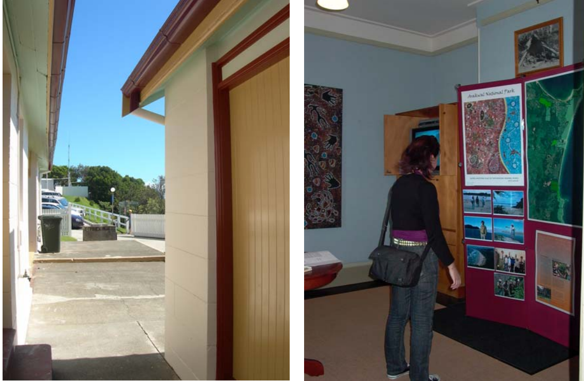
Views of the rear of the former Head Lightkeeper's quarters (left) and the cultural display in the former sitting room (right) Source: Ellsmore 2008
