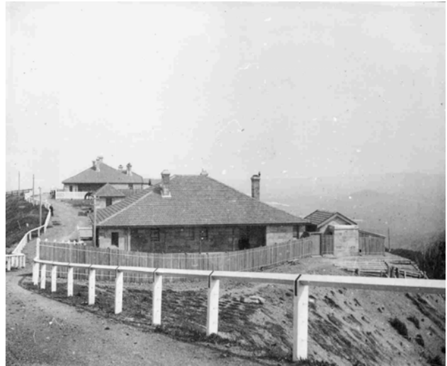
Figure 5: View looking south taken to record the finished works. Source: AONSW Reel 2643; Frame 2003, photo taken in 1902
