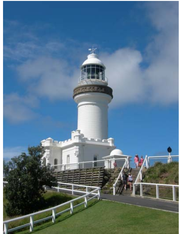
Figure 37: Cape Byron Lighthouse 2008. Source: Ellsmore 2008
