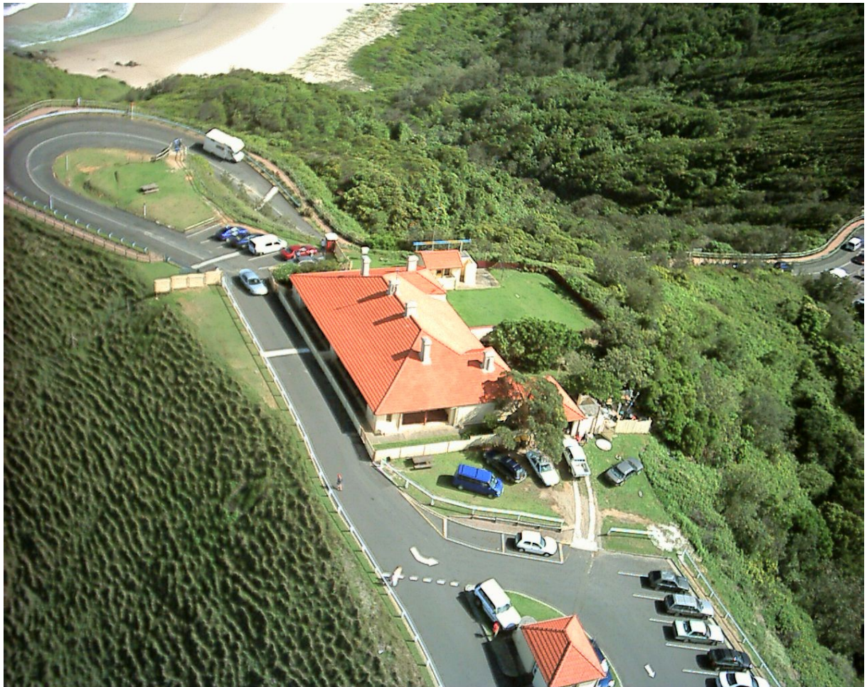
Aerial view of the southern precinct. Note the fence line which was located at the site entry (where the blue car is entering the site). Source: Ashley Wilmont c. 2003
