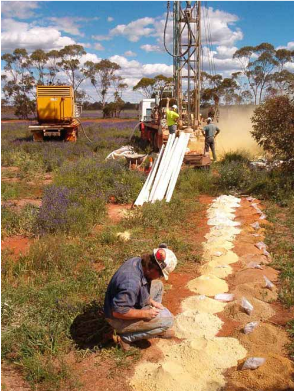
Plate 6: Drilling and sampling monitoring bores
