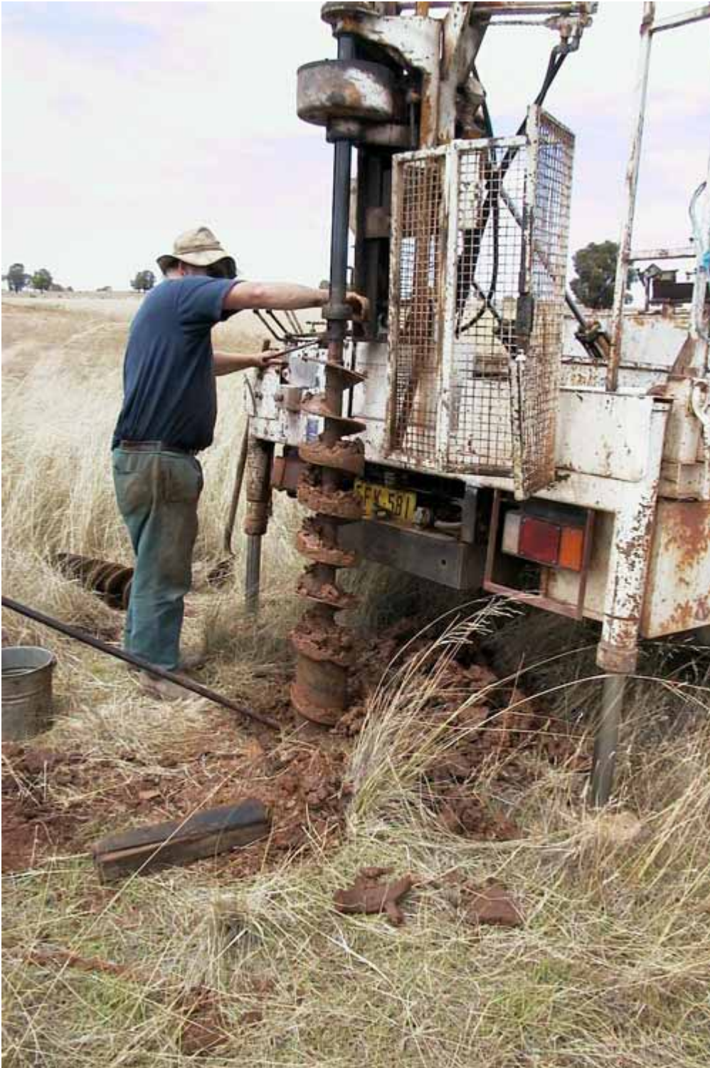
Plate 4: Auger sampling and monitoring bore installation
