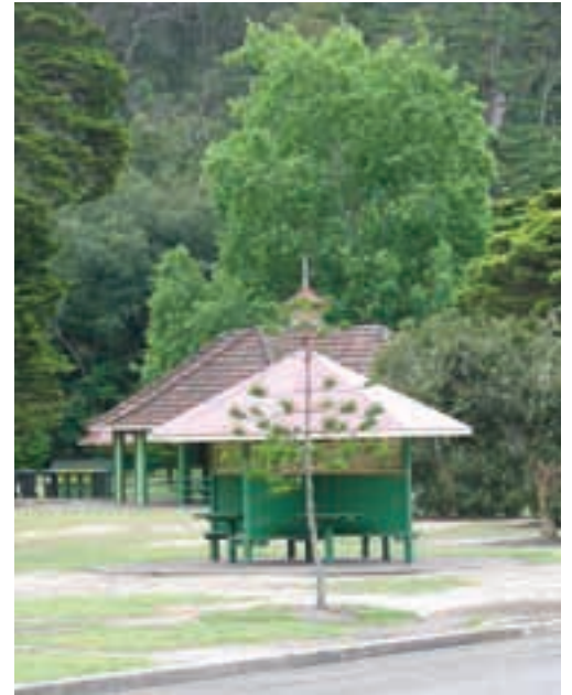
P11. Original 1930s Low Octagonal Coned Roof picnic shelter (source CM* 2006).
