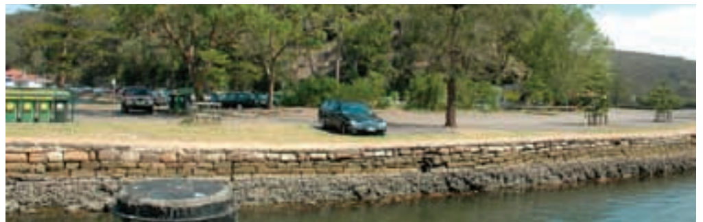
P40. The Wharf Area is currently dominated by expanses of bitumen (source: CM*)
