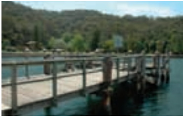
P23. The Wharf (source: CM*)
