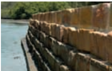
P26. Sandstone Seawall (source: CM*)
