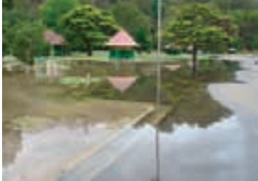
P10. Orchard Park with King-tide inundation (January 2006). (source: CM*)
