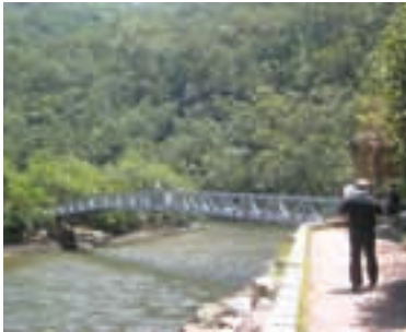
P69. Footbridge, 2006 (source: CM*)
