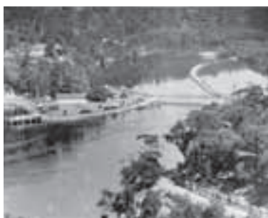
P24. Revetment wall to Gibberagong Park complete (source: NPWS Archives)
