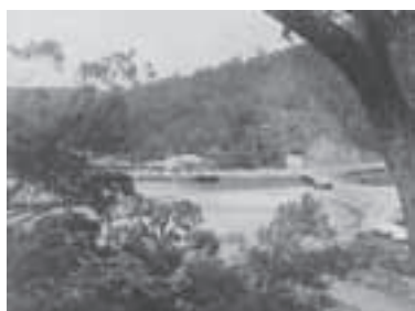
P10. Cockle Creek showing seawall to north of causeway with Wharf Area and Orchard Park South already reclaimed, while Orchard Park awaits reclamation works (Source: Hornsby Council/ No. 00192)
