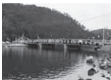
P35. Pre stressed concrete bridge across Cockle Creek, c.1956 (source: NPWS Archives)
