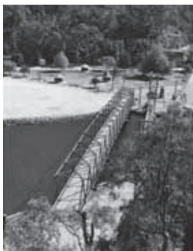
P16. The one lane Bailey bridge and adjacent footbridge across Cockle Creek. (Source: NPWS Archives)
