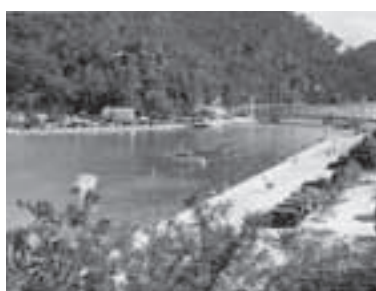
P32. Temporary military footbridge over Cockle Creek (source: NPWS Archives)
