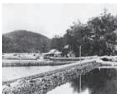
P20. Revetment walls constructed either side of Causeway on western side of Cockle Creek (source: NPWS Archives)
