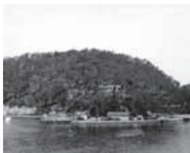
P21. Wharf Area with new jetty (source: NPWS Archives)
