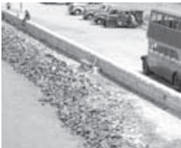
P58. Orchard Park Seawall, 1940s (source: NPW Archives)
