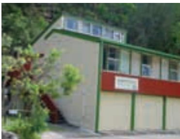
P61. Gibberagong Environmental Education Centre, South Elevation showing textured brickwork, 2006 (source: CM*)
