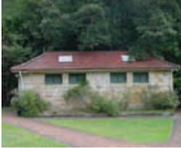
P48. Toilet Block, East Elevation, 2006 (source: CM*)
