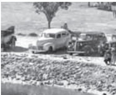
P56. Orchard Park Stone Revetment, 1930s (source: NPW Archives)
