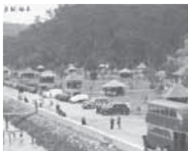
P29. New retaining wall along Orchard Park (source: State Records of NSW/ID No.12932)
