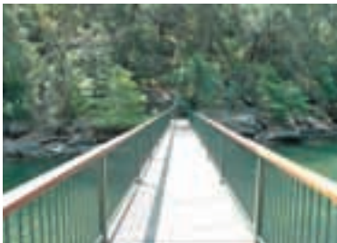
P14. Apple Tree Bay Bridge, 2006 (source: CM*)
