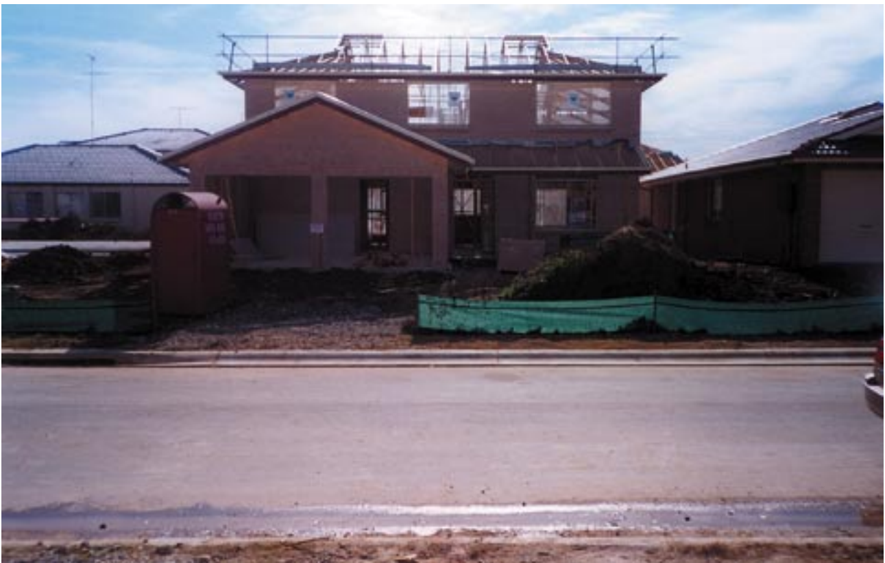
Figure 6. Sediment control measures on a construction site
