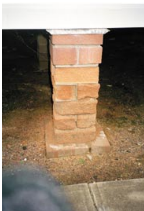
Figure 8. Effects of salinity (a) Crumbling of mortar and bricks show the effects of salinity (b) Piers affected by salinity
