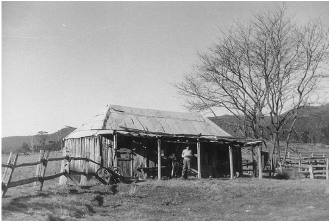
Figure 2.2. The Bendethera homestead located near the yards
