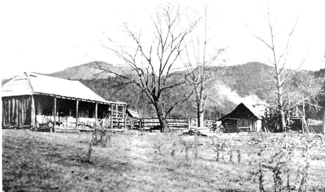
Figure 3.1 Bendethera homestead c.1910 located next to the yards with adjacent kitchen (right)
