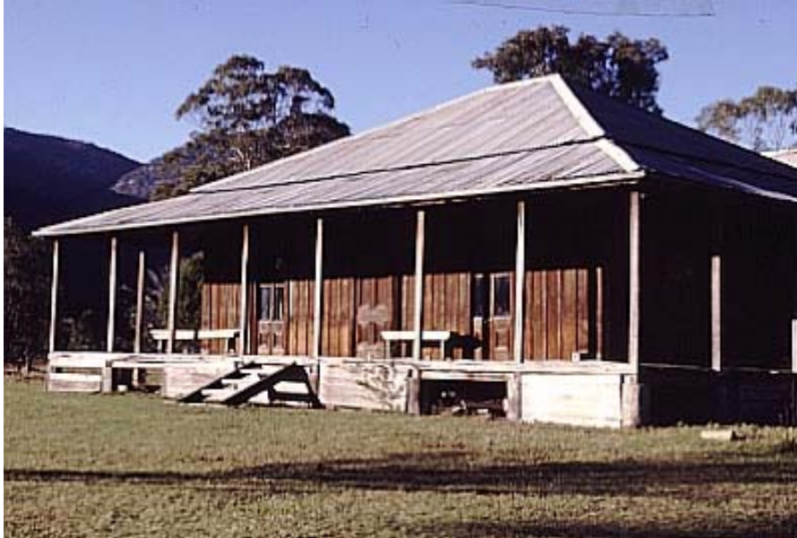
Figure 5.2 Kunderang East Pastoral Station homestead (Source: Heritage Branch, DoP)
