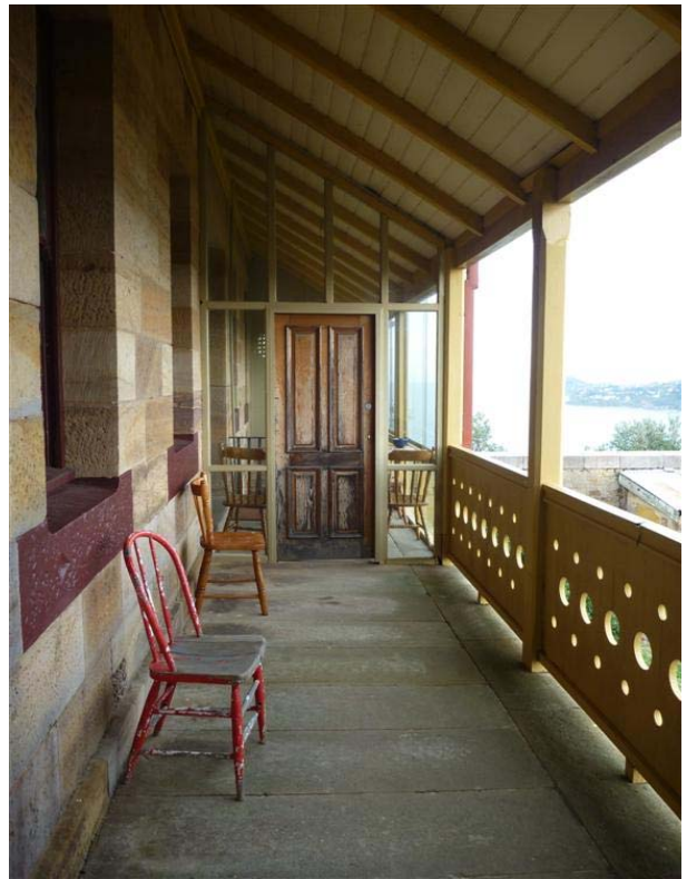
Figure 4.12 Rear verandah Head Light Keeper's Cottage (Source: GAO, 2011)
