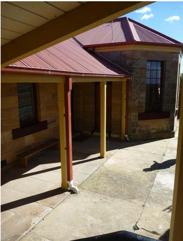
Figure 4.11 Front courtyard of Head Light Keeper's Cottage (Source: GAO, 2011)
