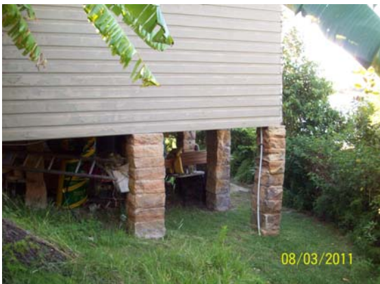
Figure 4.28 Sandstone piers (Source: GAO, 2011)
