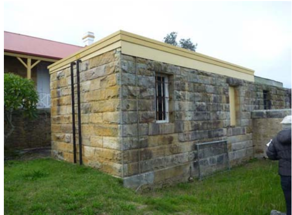
Figure 4.14 Outbuilding to northern most Assistant Light Keeper's Cottage (Source: GAO, 2011)
