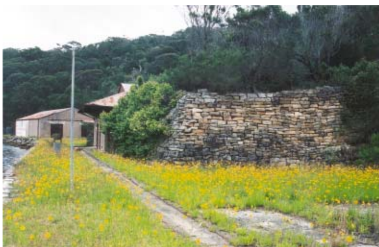
Figure 3.6.20 Stone retaining wall on concourse, with light rail track in front, 2001
