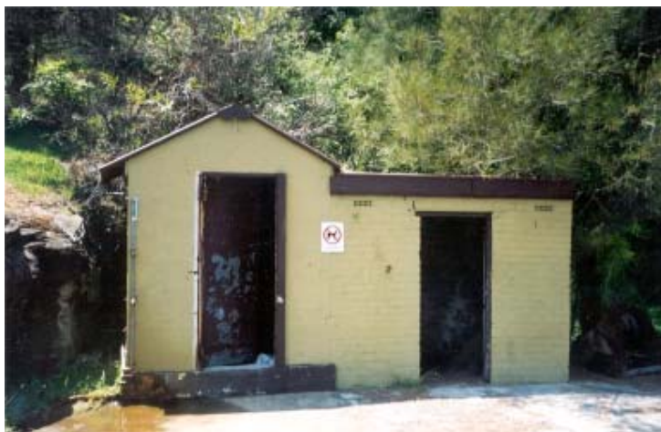
Figure 3.6.25 Original toilet structure, 2001
