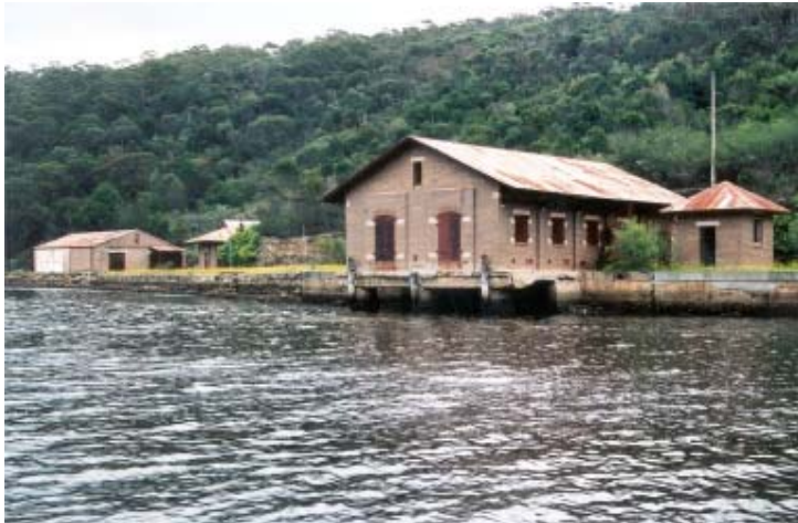
Figure 3.6.9 Receiving shed and telegraph office, including magazines No. 7 & 9, 2001
