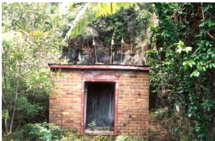
Figure 3.6.18 Detonator storage shed
