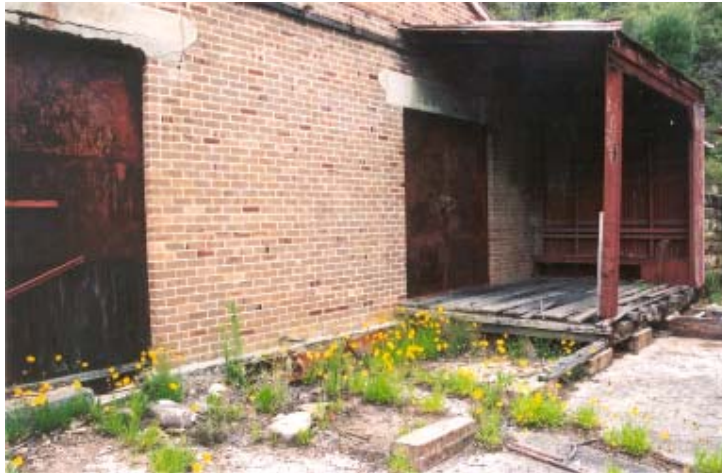
Figure 3.6.13 Partially demolished verandah to magazine No.9, 2001
