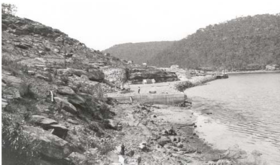
Figure 2.4.8 Site of new magazine station, Bantry Bay, c.1913. GPO1-31373, reproduced with permission, State Library of NSW.
