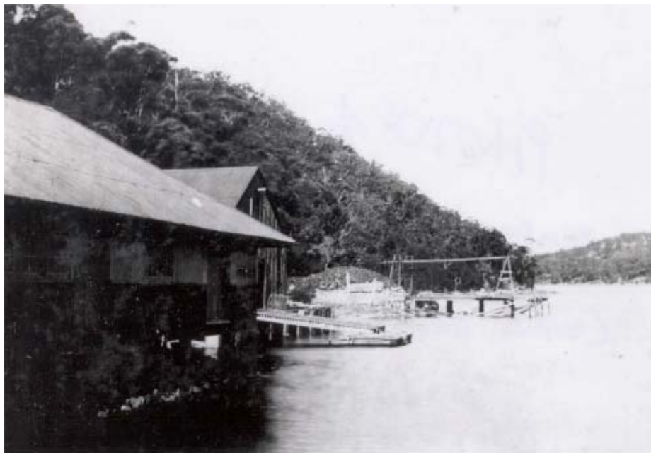
Figure 2.4.4 Proposed site of coal bunker at Bantry Bay, May 1918, GPO1-21185, reproduced with permission, State Library of NSW.
