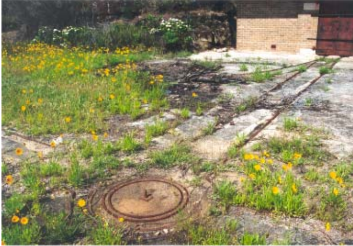
Figure 3.6.21 Concrete concourse with light rail tracks and turntable, 2001
