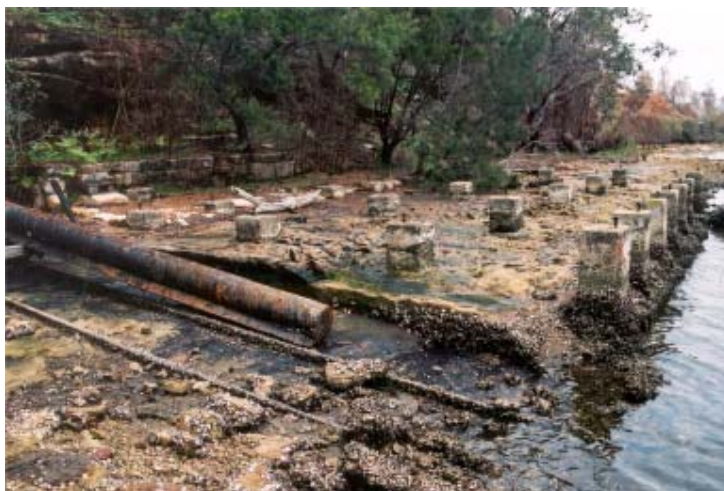
Figure 3.6.26 Slipway and stone piers of dance hall, 2001
