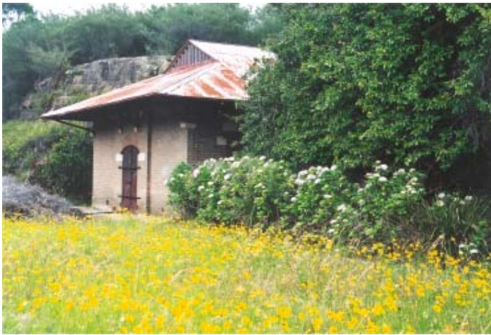
Figure 3.6.3 Magazine No.2, showing hydrangeas and weed ( Coreopsis SP) covering concourse, 2001
