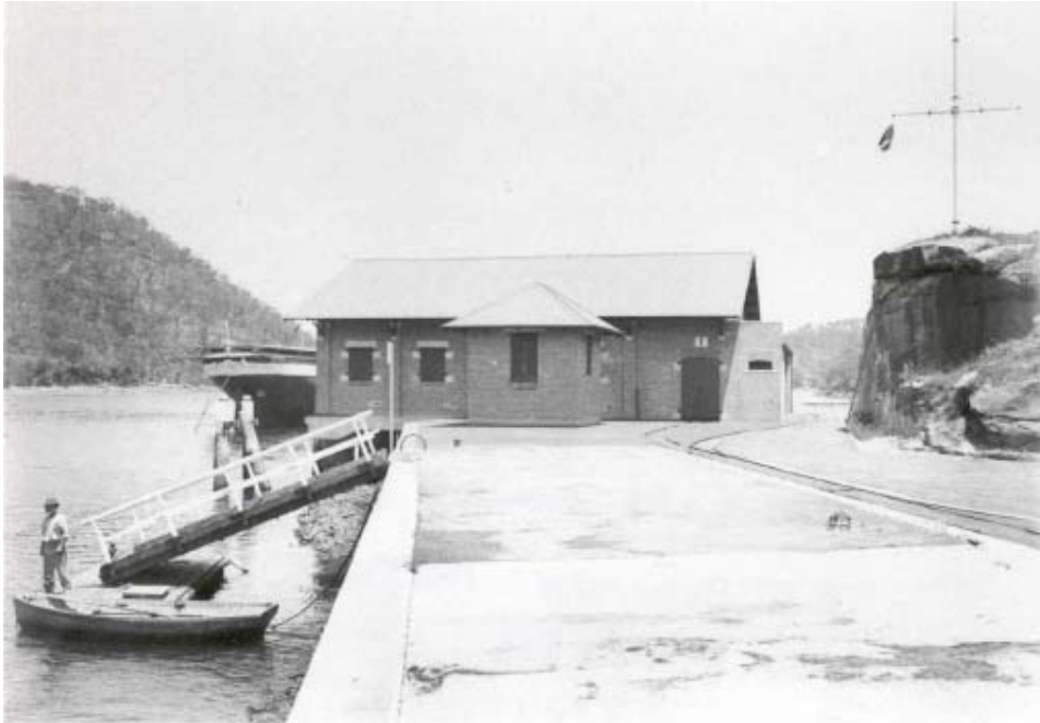
Figure 2.4.11 Receiving House, guardhouse and receiving jetty, January, 1916, GPO1-31864, reproduced with permission, State Library of NSW.
