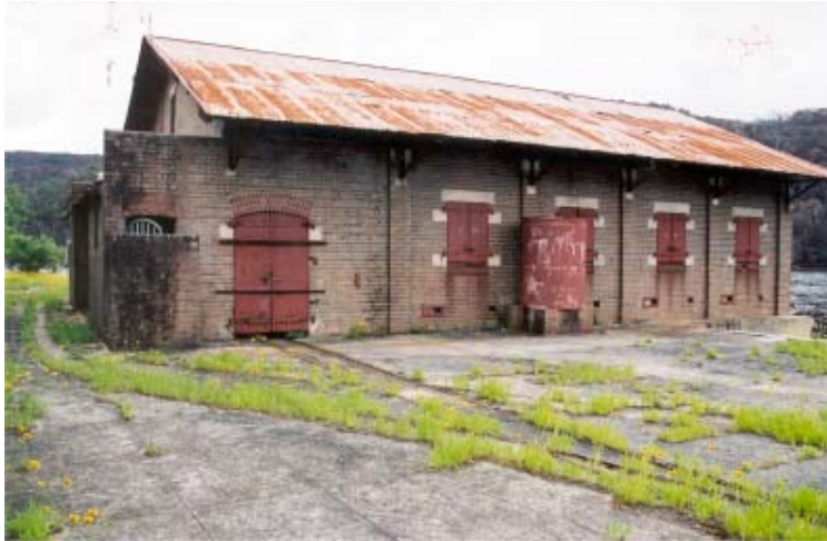
Figure 3.6.10 Detail of southern elevation of receiving shed, 2001
