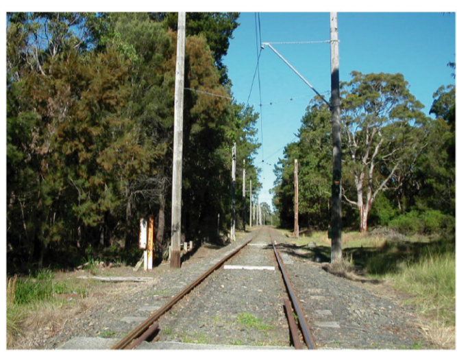
1 RAIL APPROACH FROM LOFTUS
