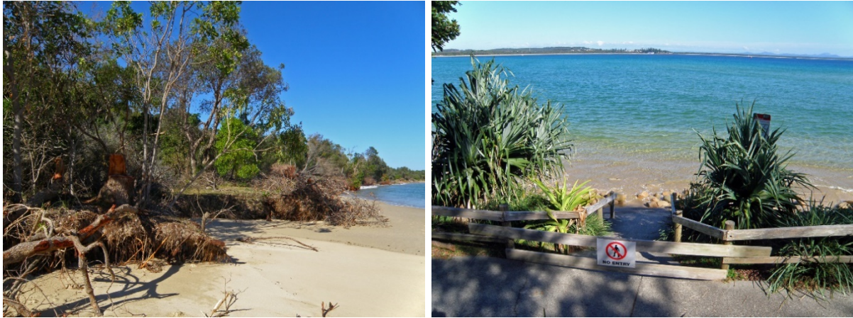
Photo 5 Beach erosion within Trial Bay Visitor Precincts has resulted in vegetation loss and the periodic closure of beach access points. Andrew Baker/DPE (2021).
