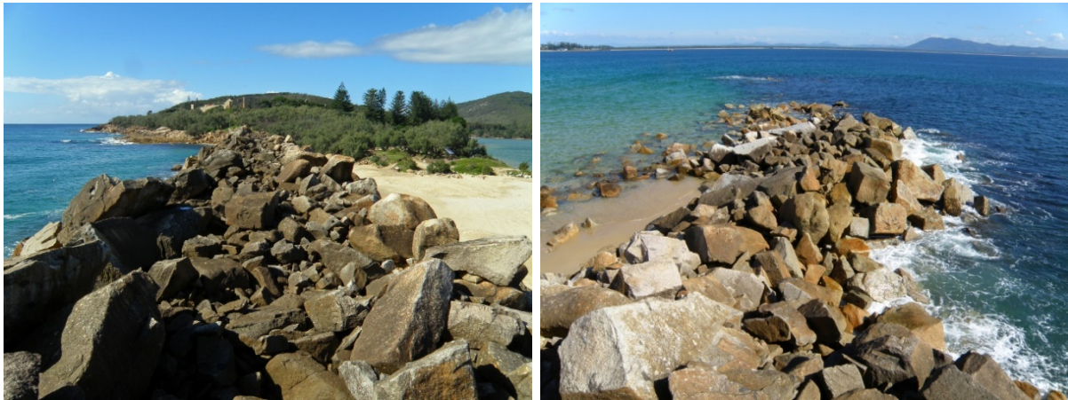
Photo 4 Laggery Point Breakwater. Andrew Baker/DPE (April 2021).
