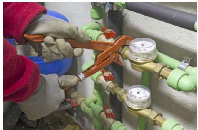
Figure 4 Plumber installing manual read water meters. (Shutterstock)
