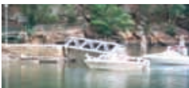
P18. Jetty and pontoon (source: CM*)
