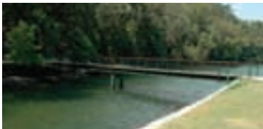
P14. Footbridge (source: CM*)
