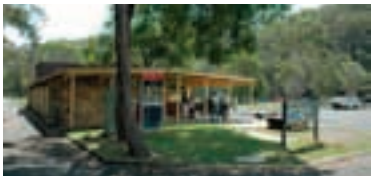
P13. Kiosk and facilities (source: CM*)
