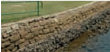
P15. Seawall (source: CM*)
