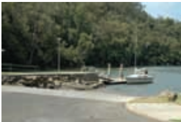
P24. Ramp at Apple Tree Bay (source: CM* 2006)
