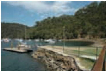
P25. Jetty, Pontoon and Boat Ramp, Apple Tree Bay (source: CM* 2006)
