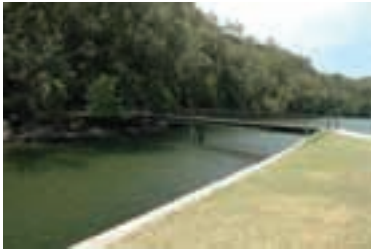
P19. Footbridge Crossing Apple Tree Creek, view looking north (source CM+ 2006)
