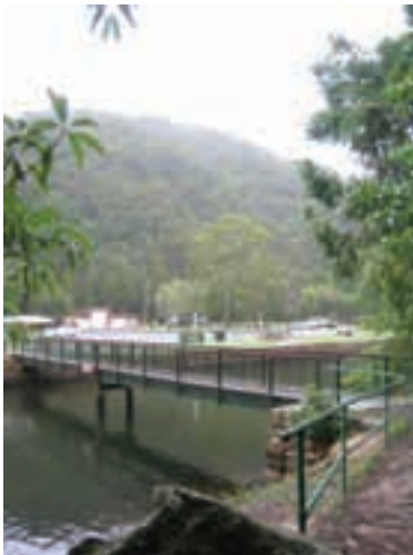
P20. Footbridge Crossing Apple Tree Creek, view looking south-west (source CM+ 2006)
