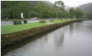
P23. Seawall on Apple Tree Bay (source: CM* 2006)
