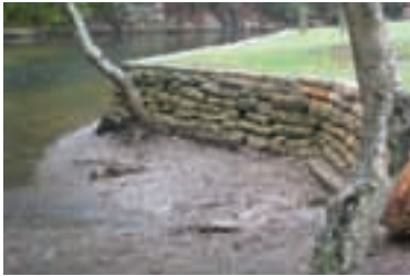
P22. Seawall, Apple Tree Bay (source: CM* 2006)
