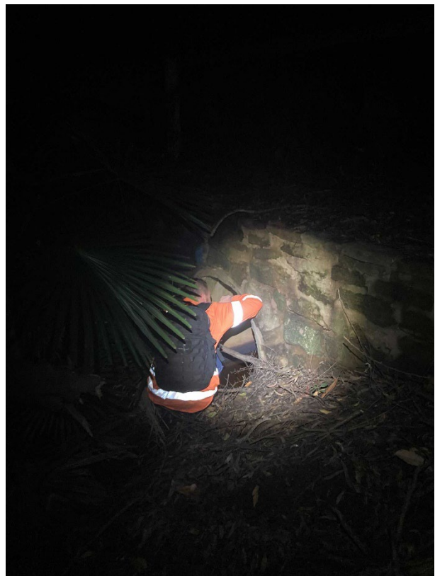
Figure 6: Culvert in figure 2
