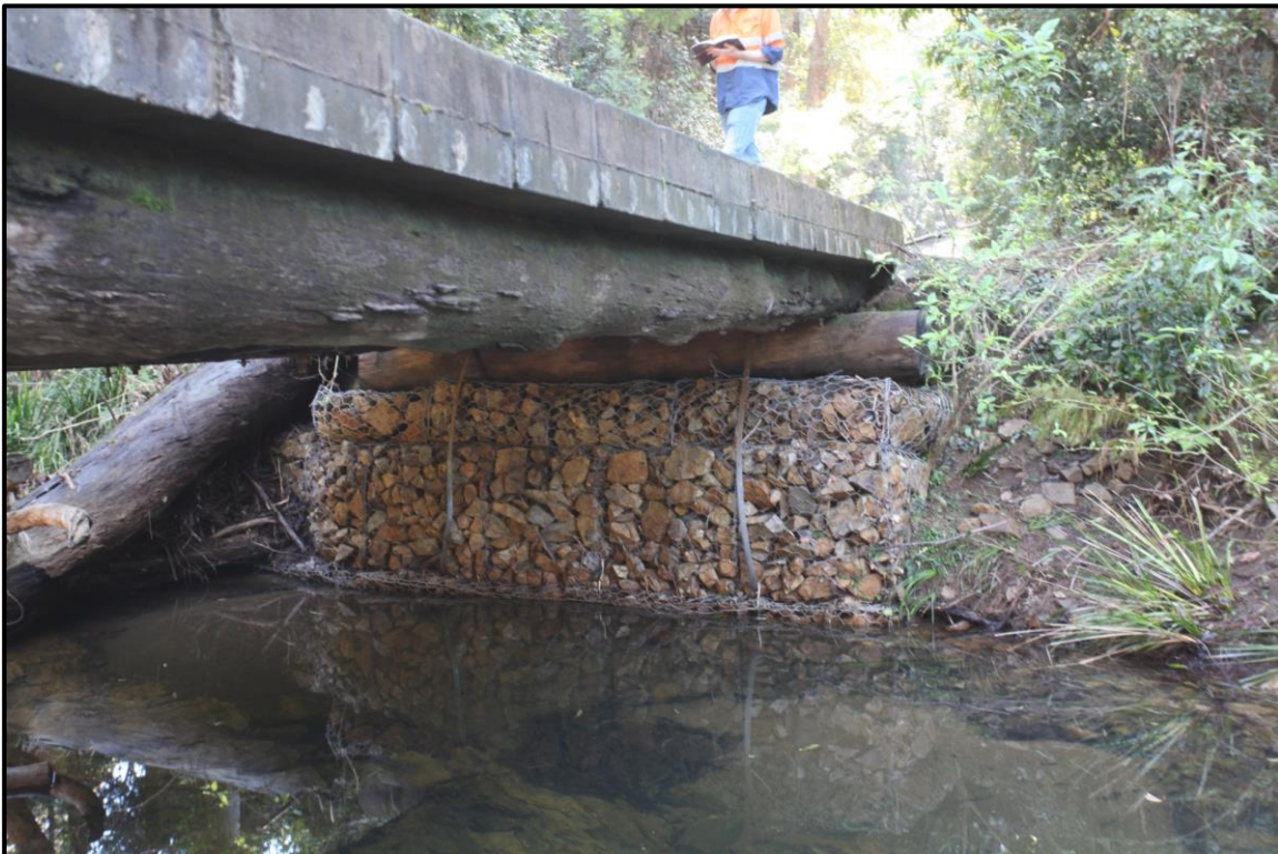
Figure 4: Budds Crossing Road Bridge replacement gabion abutment, facing north.
