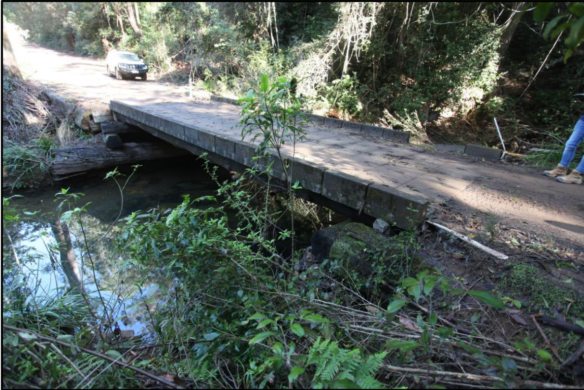
Figure 3: Budds Crossing Road Bridge facing southwest.
