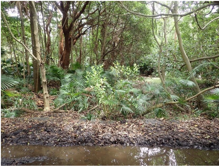
Figure 56. View north along piped section of creek existing track and culvert.
