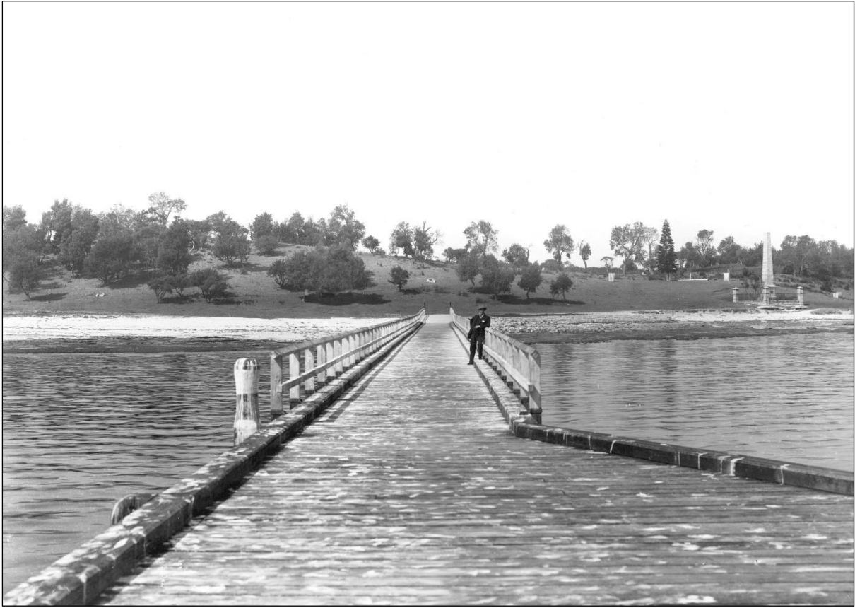
Figure 12. View south in 1905 to the newly constructed wharf and Cook Monument on the right.
