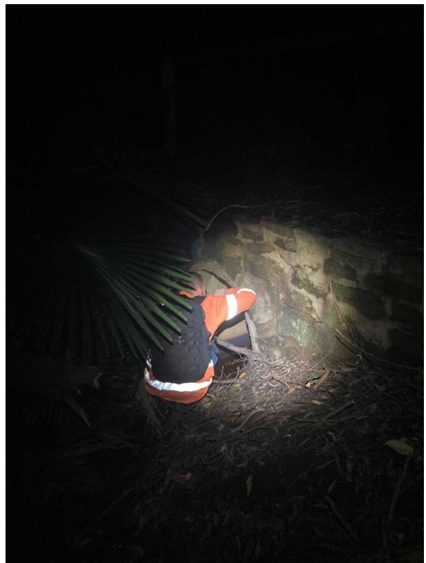
Figure 6: Culvert in figure 2
