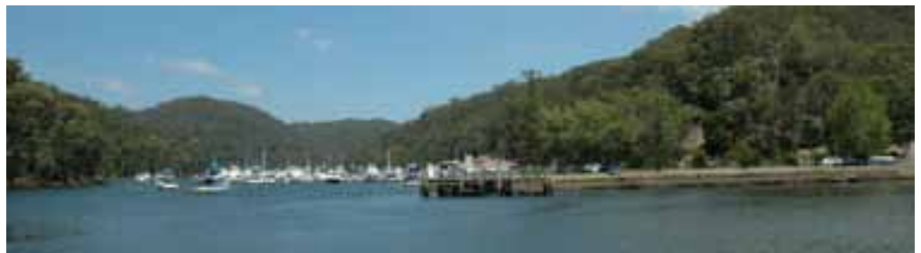
Sandstone Seawall at Bobbin head
