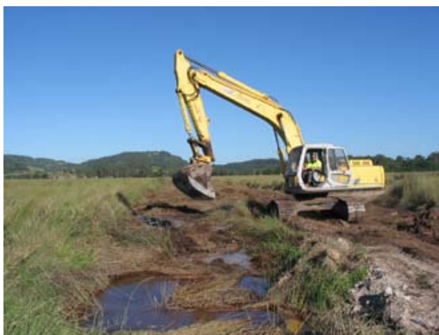
Plate 10. Drain infilling at Cudgen
