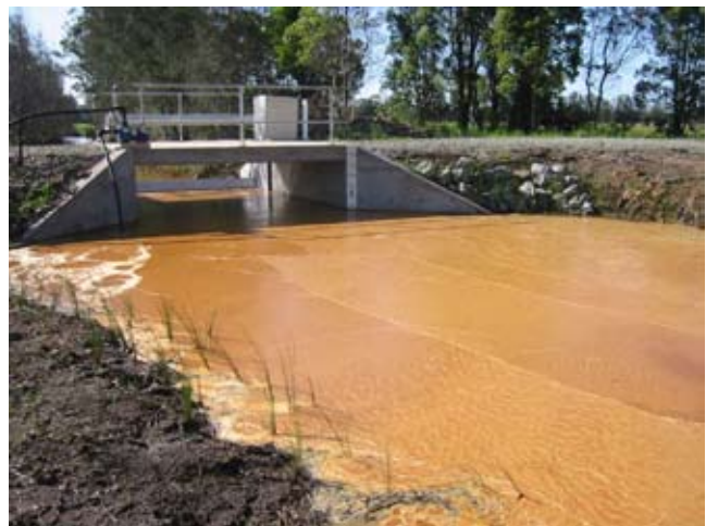
Plate 5. Iron floc caused by liming with hydrated lime at Partridge Creek on the Hastings
