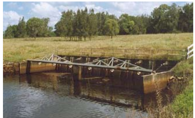
b) Lifting devices at Rocky Mouth Creek on the Richmond attached to a side-mounted winch by a gantry
