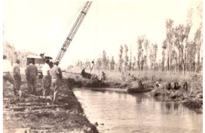
Plate 1. Drainage works on the Macleay River floodplain in 1963
