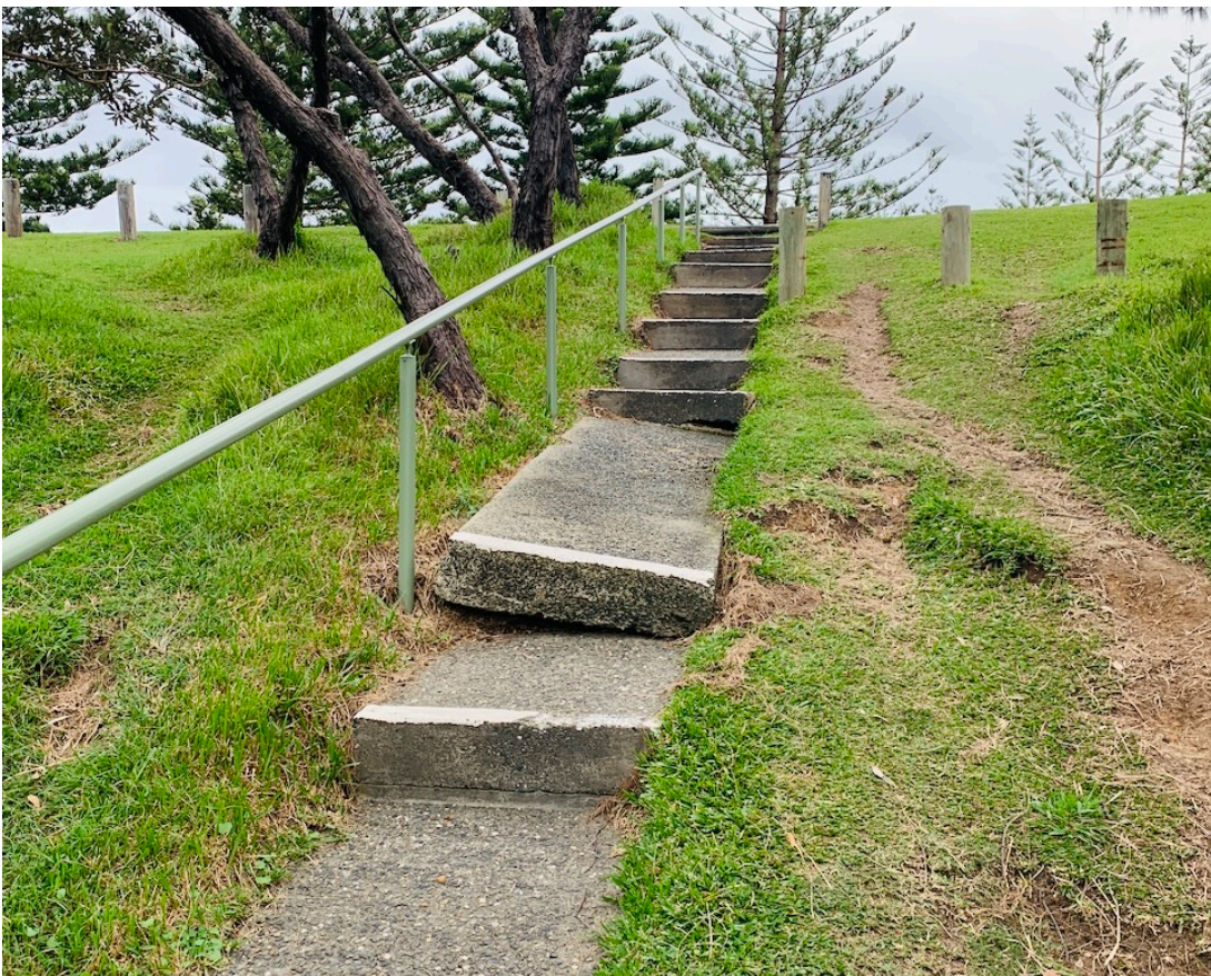
FIGURE 85: EXISTING STEPS (ITEM 4.24)
