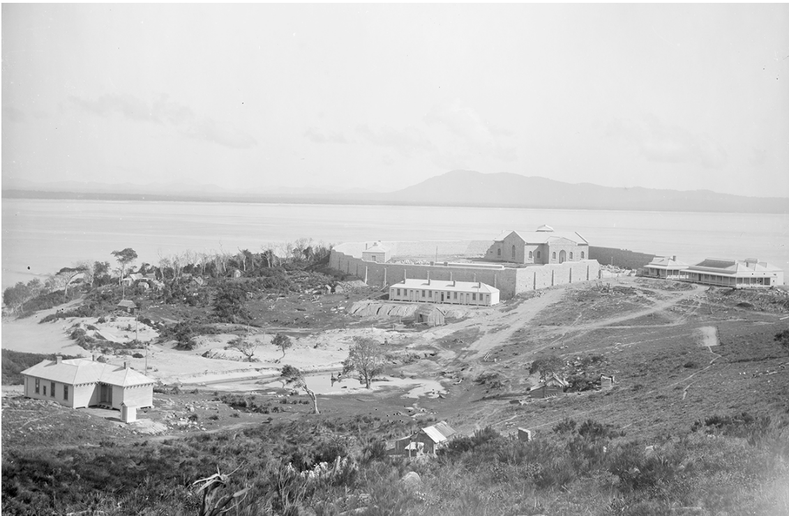
FIGURE 9: PHOTOGRAPH OF TRIAL BAY GAOL UNDER CONSTRUCTION (C.1880S)
