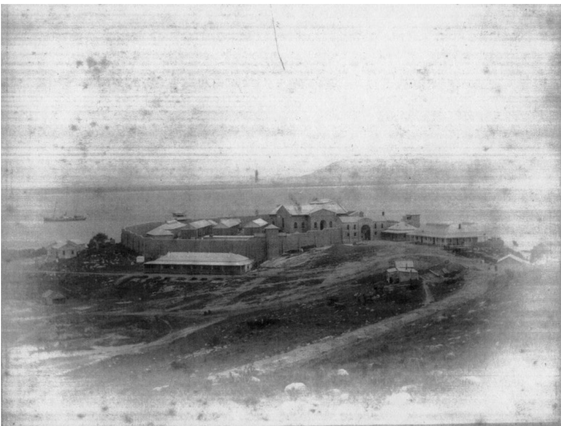
FIGURE 10: PHOTOGRAPH OF TRIAL BAY GAOL UNDER CONSTRUCTION (PRE-1889)
