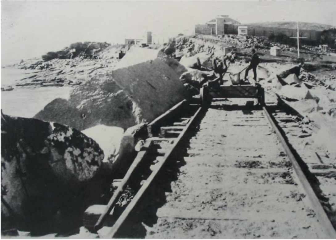
FIGURE 19: TRIAL BAY BREAKWATER TRAMWAY
