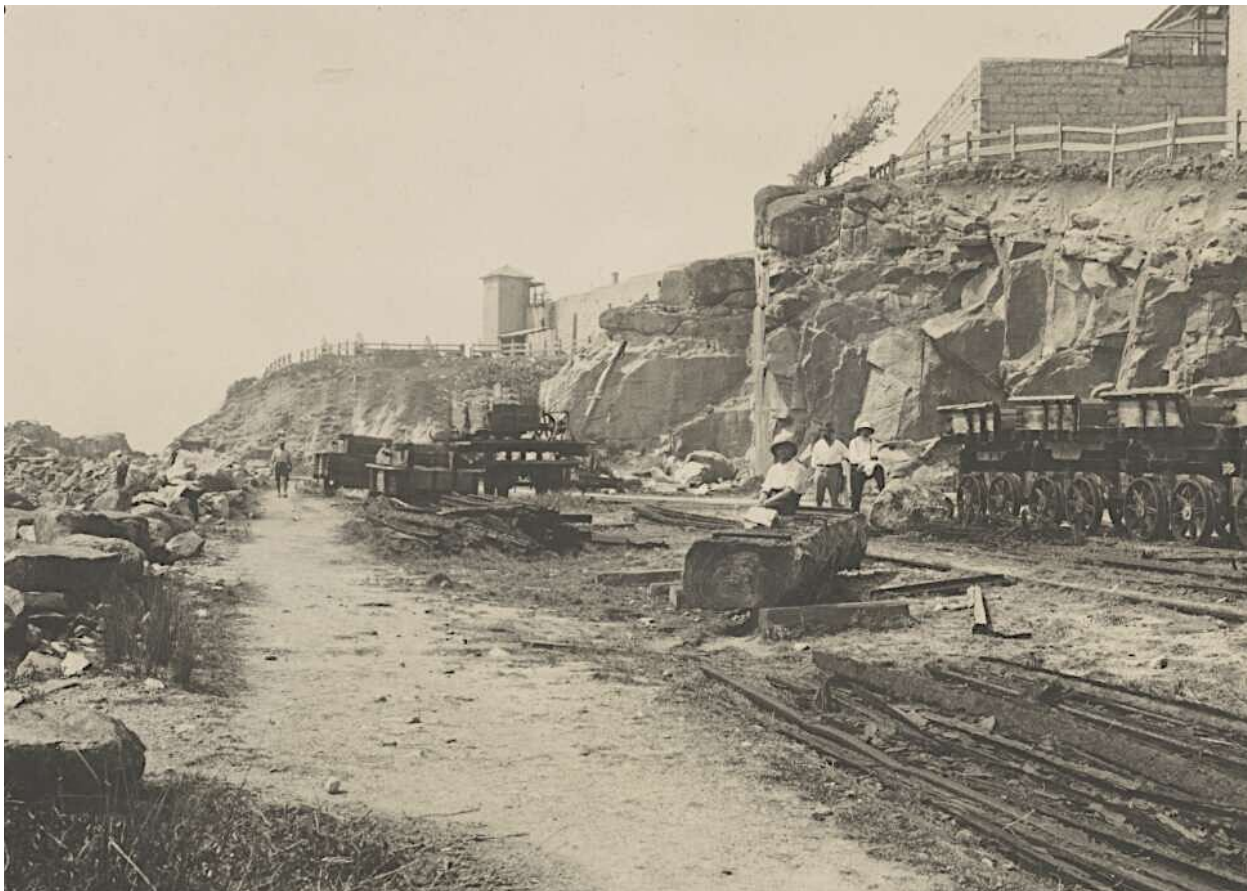
FIGURE 26: RAILWAY DUMP CARS ON THE BREAKWATER AT TRIAL BAY (1917)
