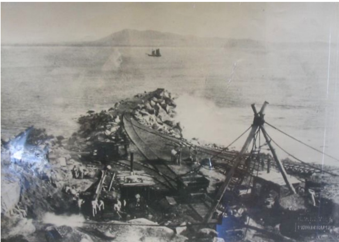
FIGURE 20: TRIAL BAY BREAKWATER CONSTRUCTION (ND)
