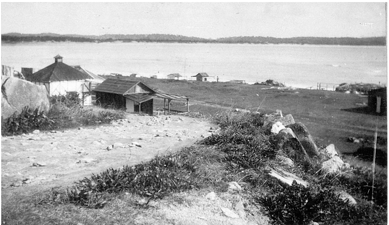
FIGURE 24: WARTIME HUTS AND STRUCTURES NEAR THE BEACH FRONT AT TRIAL BAY (1915-1917)
