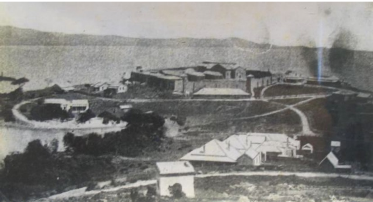
FIGURE 12: PHOTOGRAPH OF TRIAL BAY GAOL FROM MONUMENT HILL (ND)
