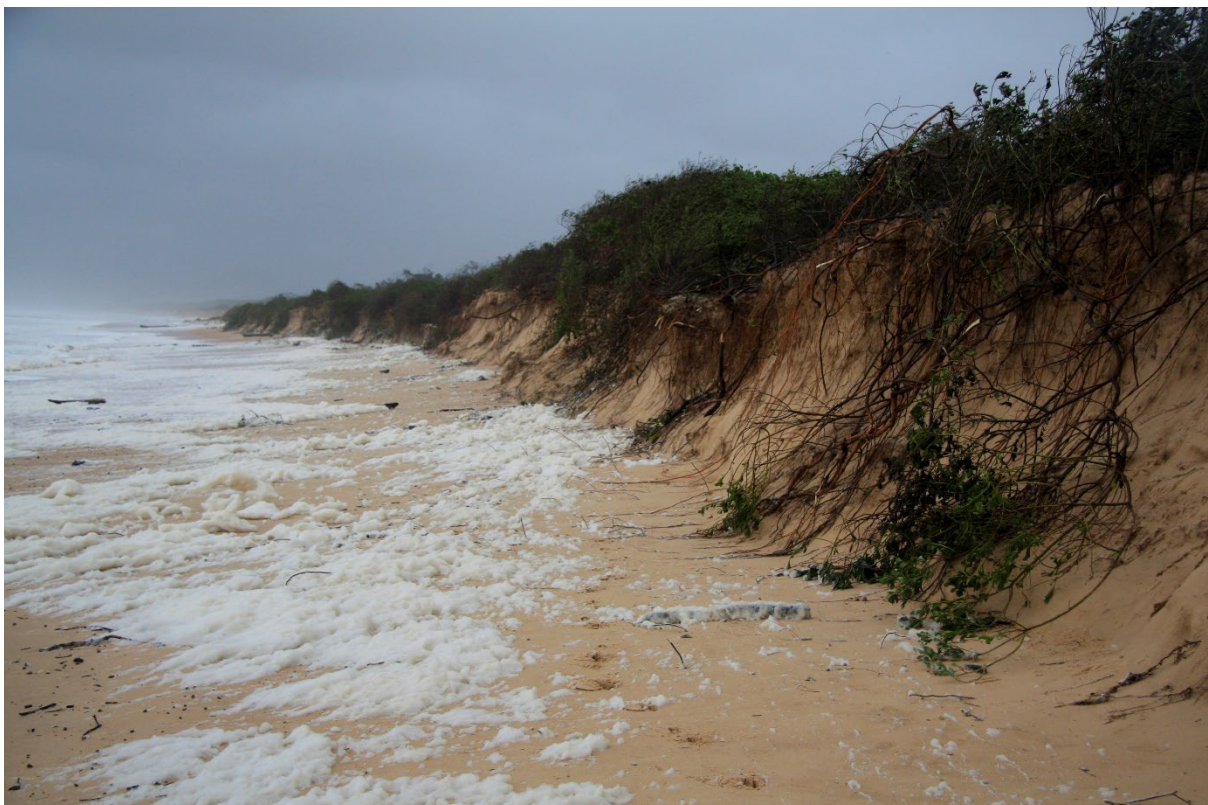
Coastal erosion from storm surges. J Turbill/DCCEEW
